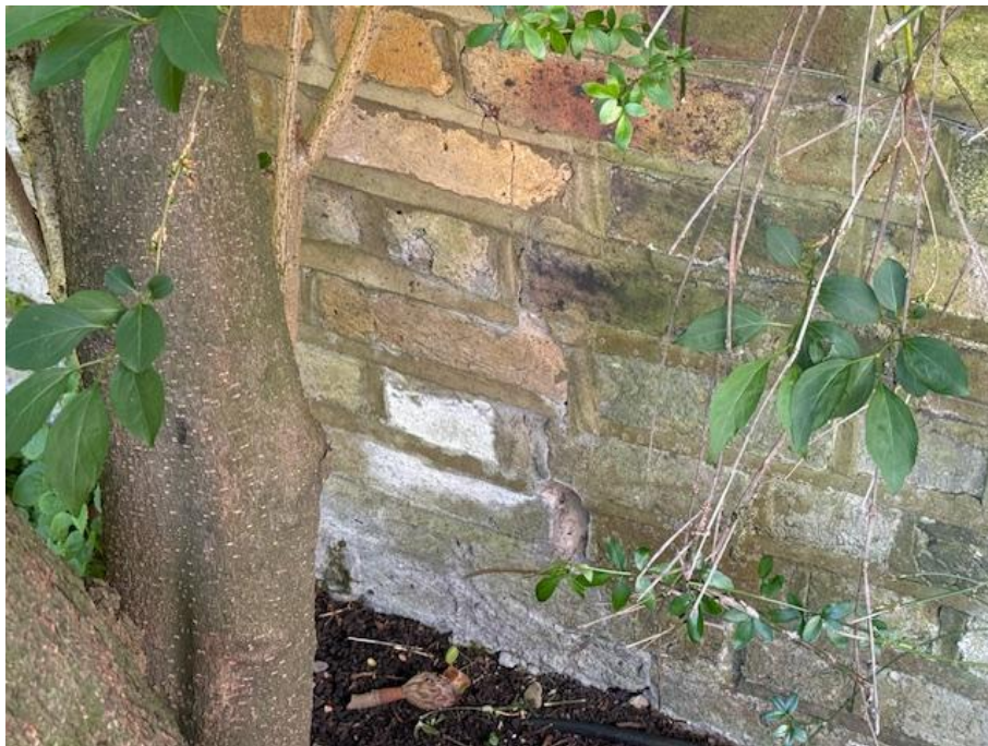
Photo 2. Previous repairs to the boundary wall adjacent to T5, with further cracking indicating tree root encroachment.
