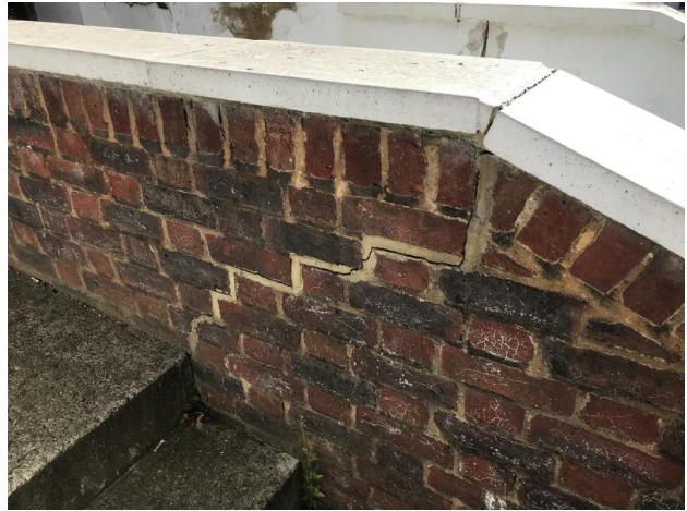
Photo 14 - Crack to boundary wall RH side
