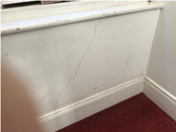
Photo 27 - Crack below window
