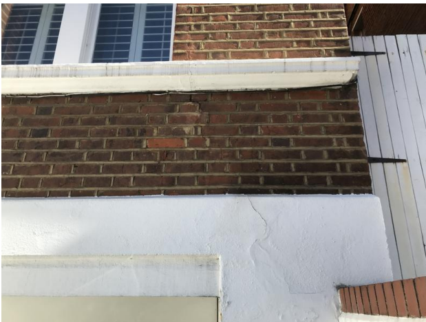
Photo 5 - Minor crack to render and bricks
