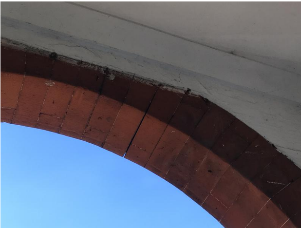
Photo 9 - Crack to arch
