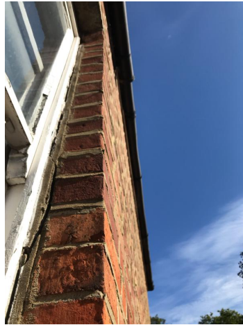
Photo 20 - Reveal pulling out
