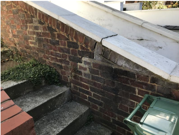
Photo 15 - Crack to boundary wall near street
