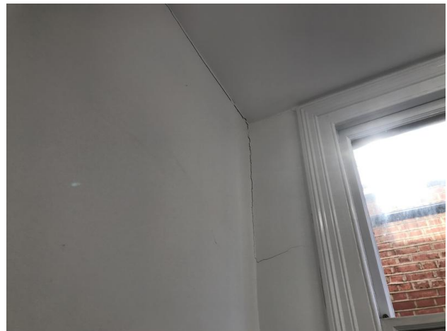
Photo 26 - Crack up to ceiling 4mm
