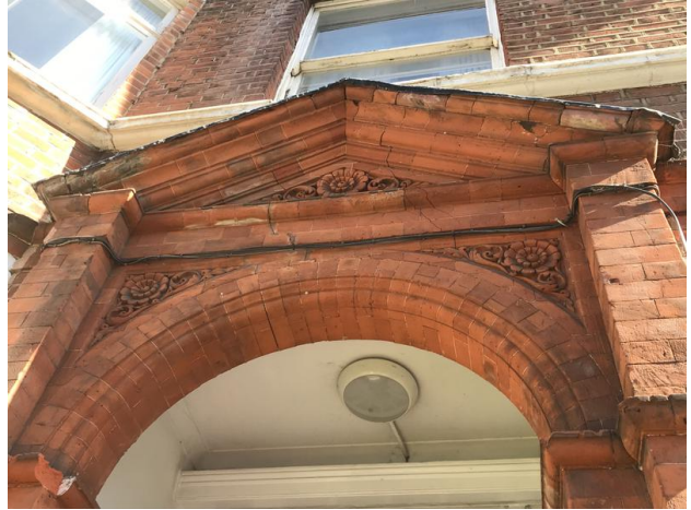
Photo 8 - Crack to decoarative portico
