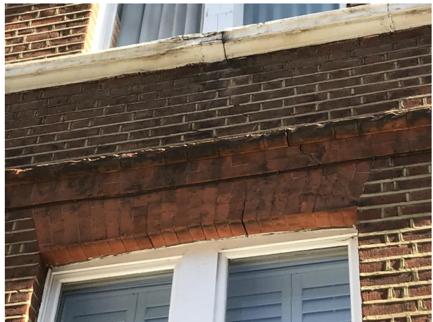
Photo 6 - Crack to brick arch
