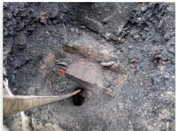
Fig 2.2: Trial Hole 2 Footing
