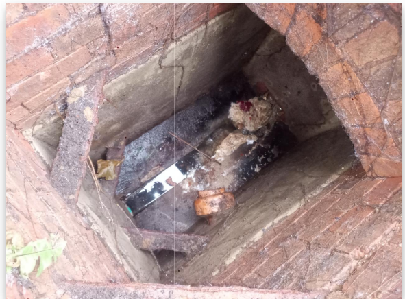
Fig 4.4: MH2 blocked, now clear
