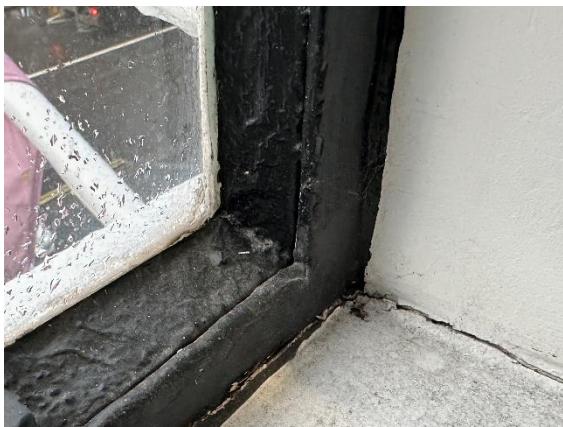
Photo 27 – Overpainted degraded putty sealant
