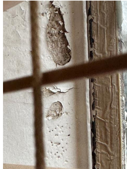
Photo 36 – Deterioration of the internal finishes due to water ingress and condensation
