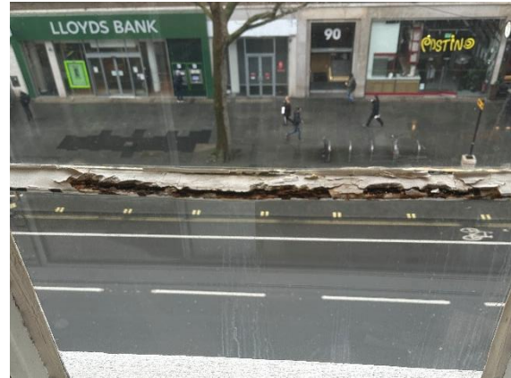
Photo 26 – Extreme degradation of the putty sealant and corrosion of the steel substrate
