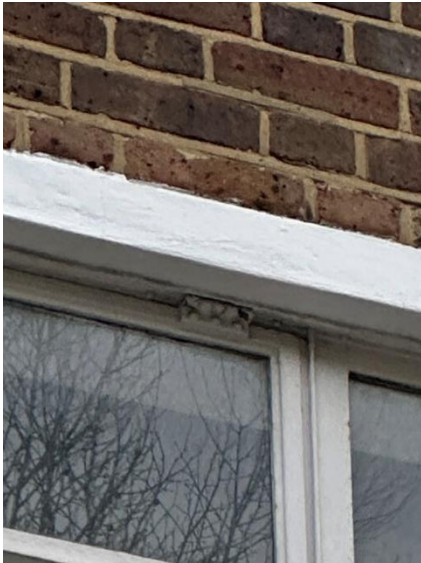
Photo 13 – Top hung window hinge
