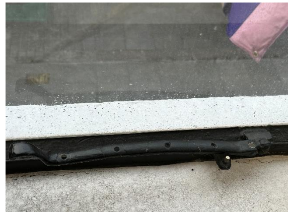
Photo 16 – Casement stay to a hinged window
