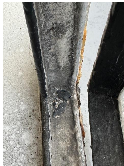
Photo 30 – Profile finish deterioration and corrosion of the steel substrate
