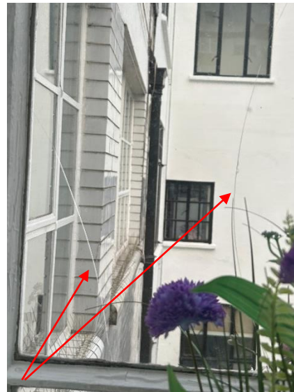
Photo 20 – Broken glazing
