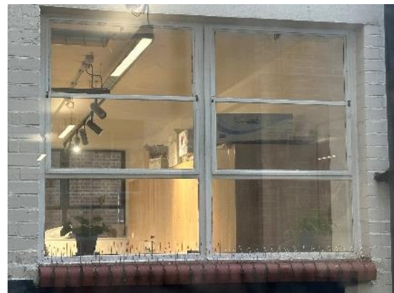
Photo 8 – Typical external view of centre pivot windows
