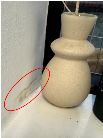
Photo 33 – Water staining to internal finishes
