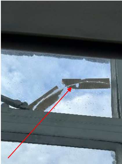
Photo 17 – Broken glazing
