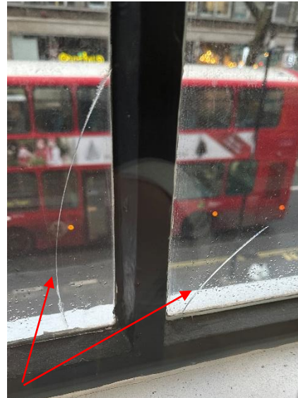
Photo 18 – Broken glazing
