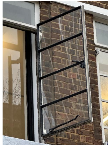
Photo 12 – Typical external view of a side hung window
