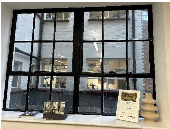
Photo 7 – Typical internal view of centre pivot windows
