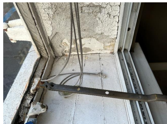
Photo 34 – Deterioration of the internal finishes due to water ingress and condensation
