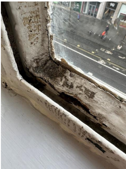
Photo 23 – Degradation of the putty sealant
