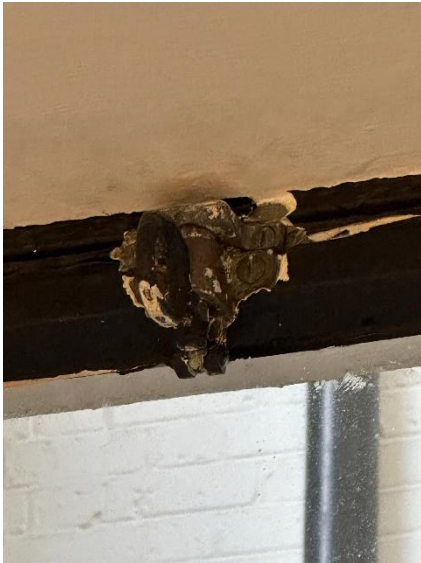
Photo 31 – Internal finishes flaked away, exposing the steel substrate
