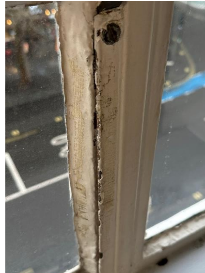
Photo 32 – Profile finish deterioration and corrosion of the steel substrate
