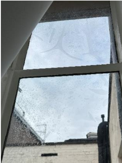
Photo 21 – Delaminated glazing film
