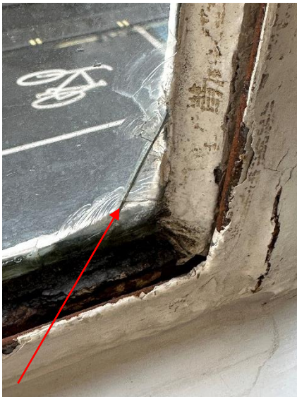
Photo 19 – Broken glazing
