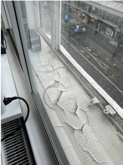
Photo 35 – Deterioration of the internal finishes due to water ingress and condensation
