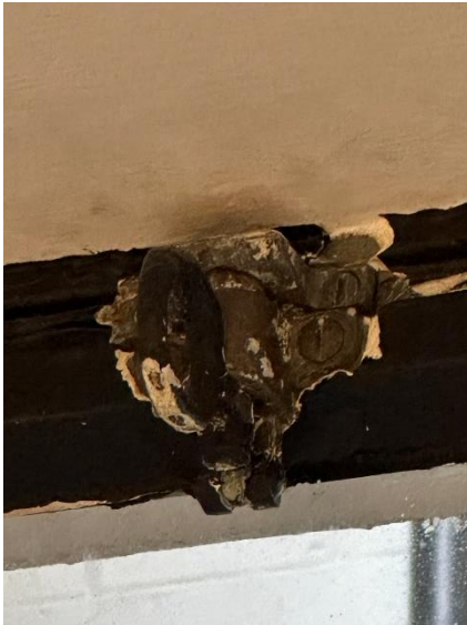
Photo 9 – Centre pivot window spring latch
