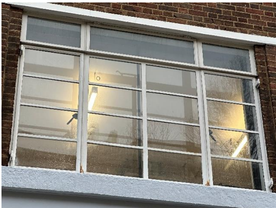
Photo 11 – Typical external view of top and side hung windows
