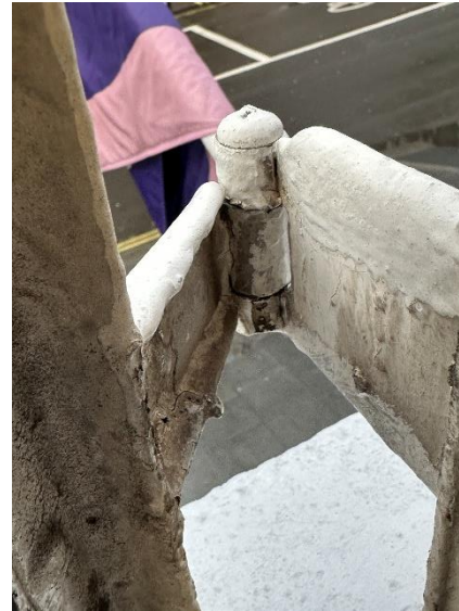
Photo 14 – Side hung window hinge
