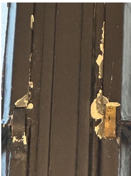
Photo 29 – Internal finishes flaked away, exposing the steel substrate
