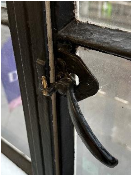
Photo 15 – Cockspur handle to a hinged window
