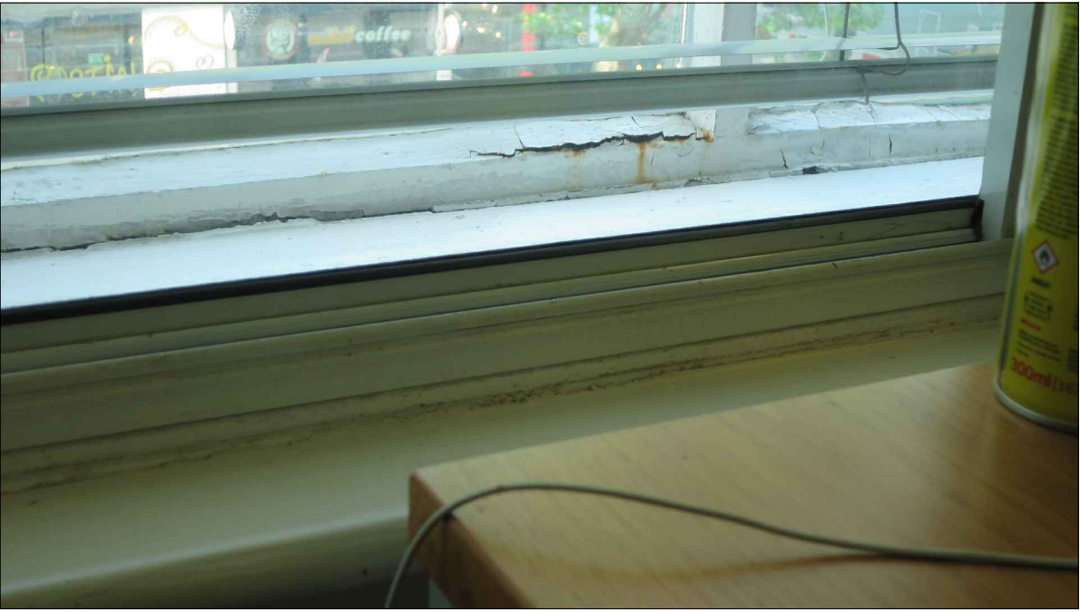
DAMAGE TO EXISTING WINDOWS
