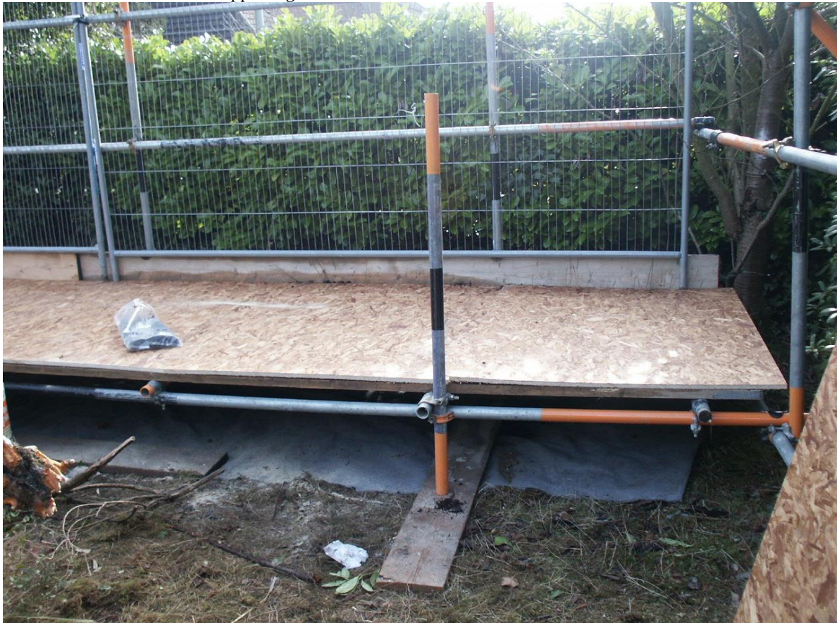
Photo 2 Scaffold framework supporting wooden boards
