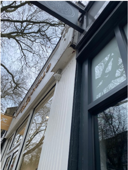
Existing right pillar high level rot
