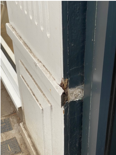
Existing right pillar low level rot
