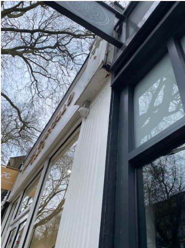
Existing right pillar high level rot
