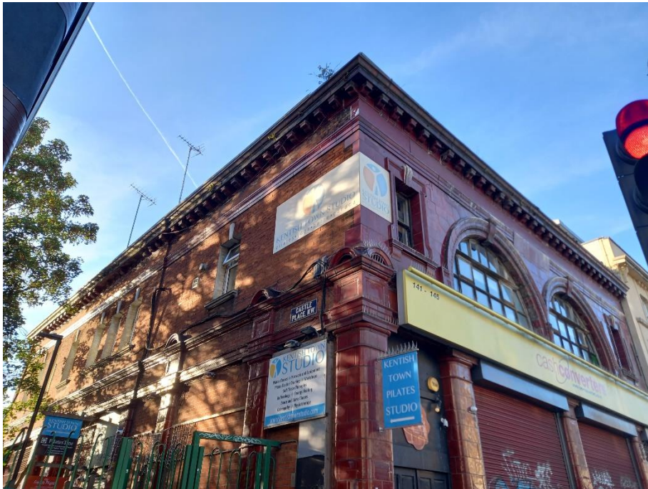
Figure 7: Brick return with Faience just to front and corner [© SKARCHITECTS]
