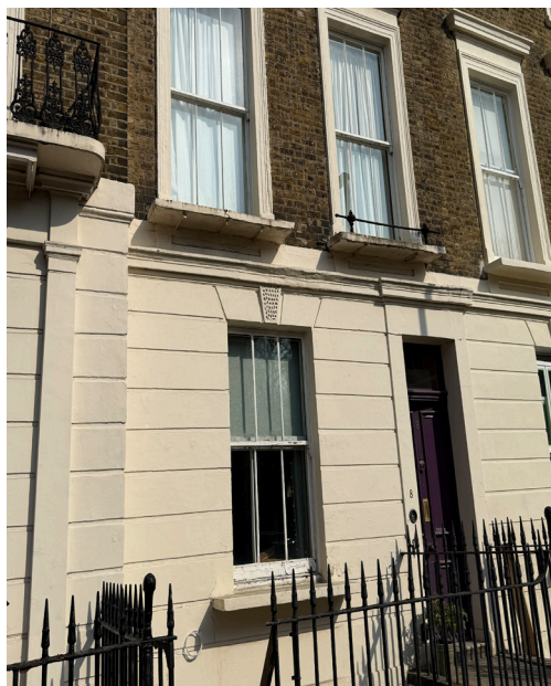
Existing render to be repaired and redecorated
