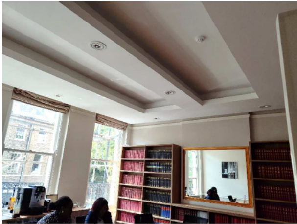
Plate 35 Showing modern suspended ceiling to front room of No. 54.
