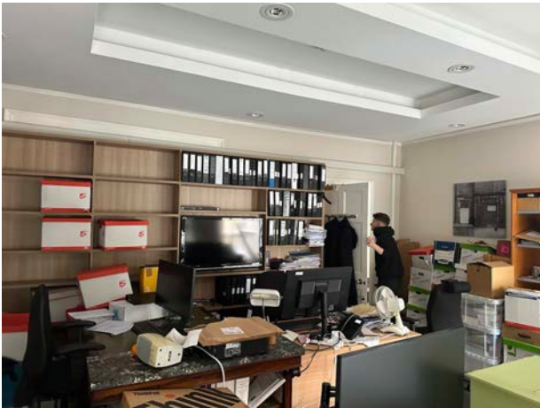
Plate 29 First floor front room of No. 53 showing suspended ceiling and obscured double door in spine wall.
