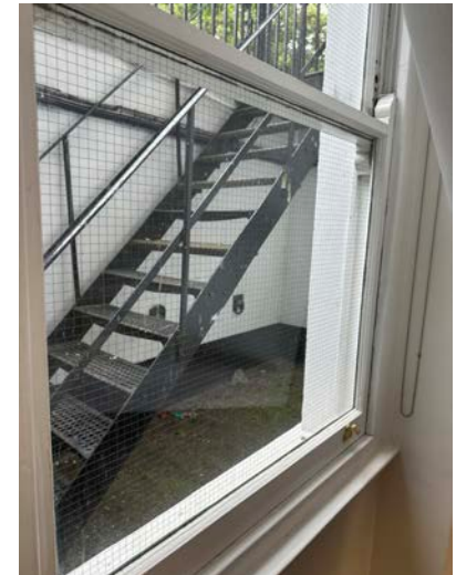
Plate 10 Modern Georgian wired glass to later window.
