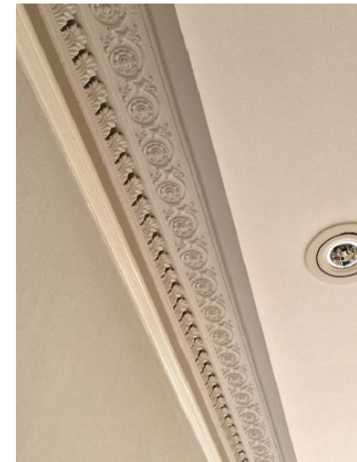
Plate 37 Modern replica cornice based on historic detail (ref: plate 30)
