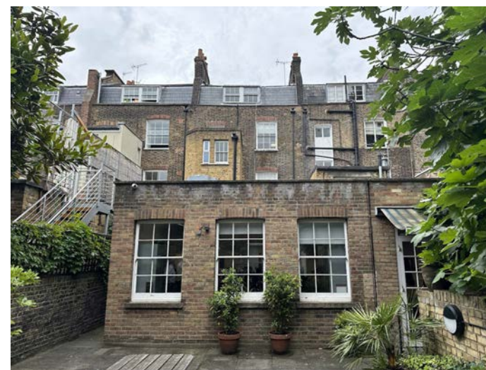
Plate 2 Rear elevation showing 1980s extension to foreground and later closet wing visible. All windows visible to this elevation are modern.
