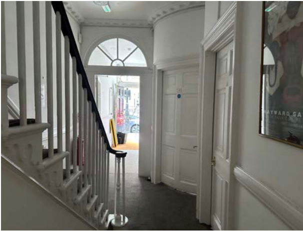
Plate 9 View towards front door showing historic joinery, open string stair and modern secondary door with fanlight to entrance.
