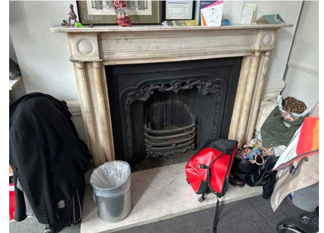
Plate 16 Historic marble fireplace with coupled engaged columns and cast iron grate.
