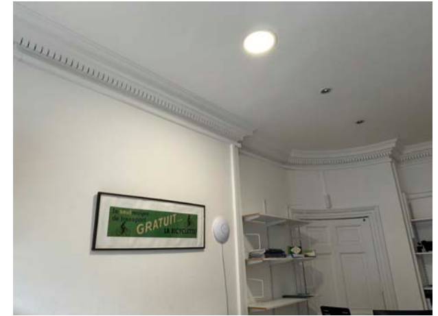
Plate 11 View of front room showing 20th century dentil cornice
