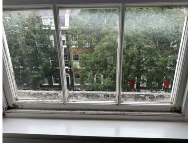
Plate 26 Detailed view of three over three sash.
