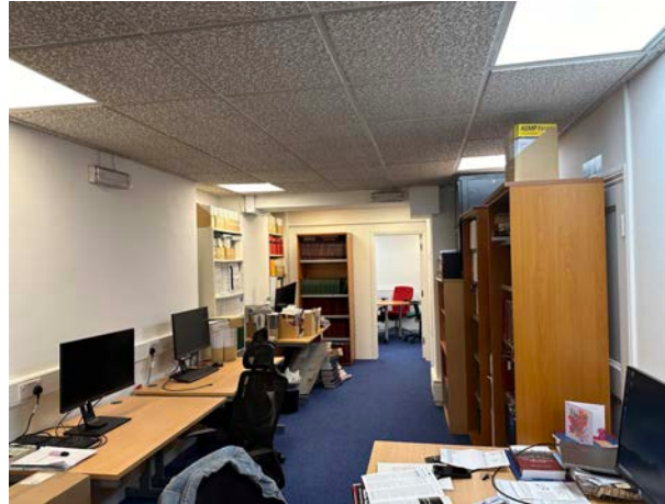
Plate 4 View looking towards rear room showing loss of spine wall and visible suspended ceiling.
