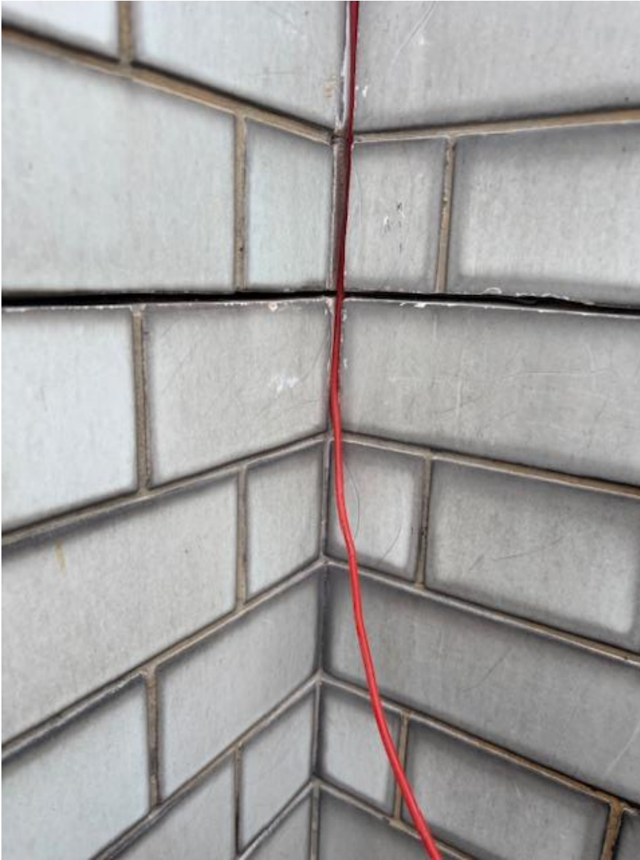
Photo 4. CP ribbon being installed to corner vertical joint.
