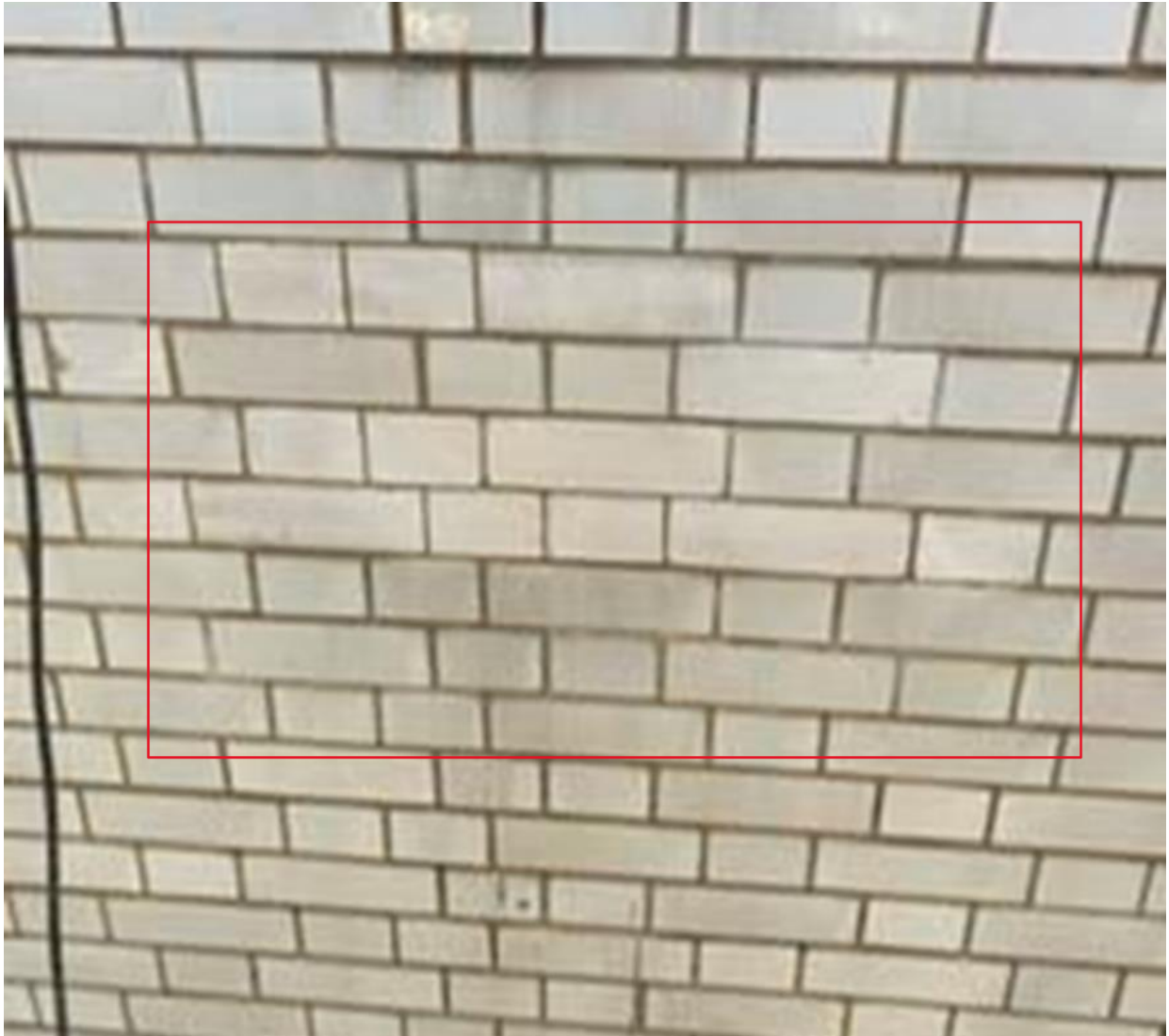
Photo 2. Reinstated brickwork repair.
