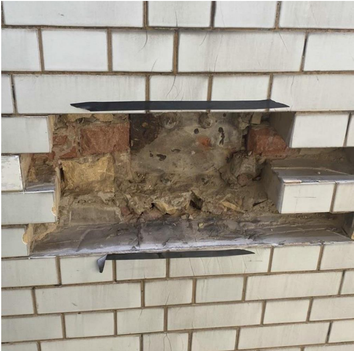
Photo 1. Existing brickwork opened up to investigate corroded steelwork.
