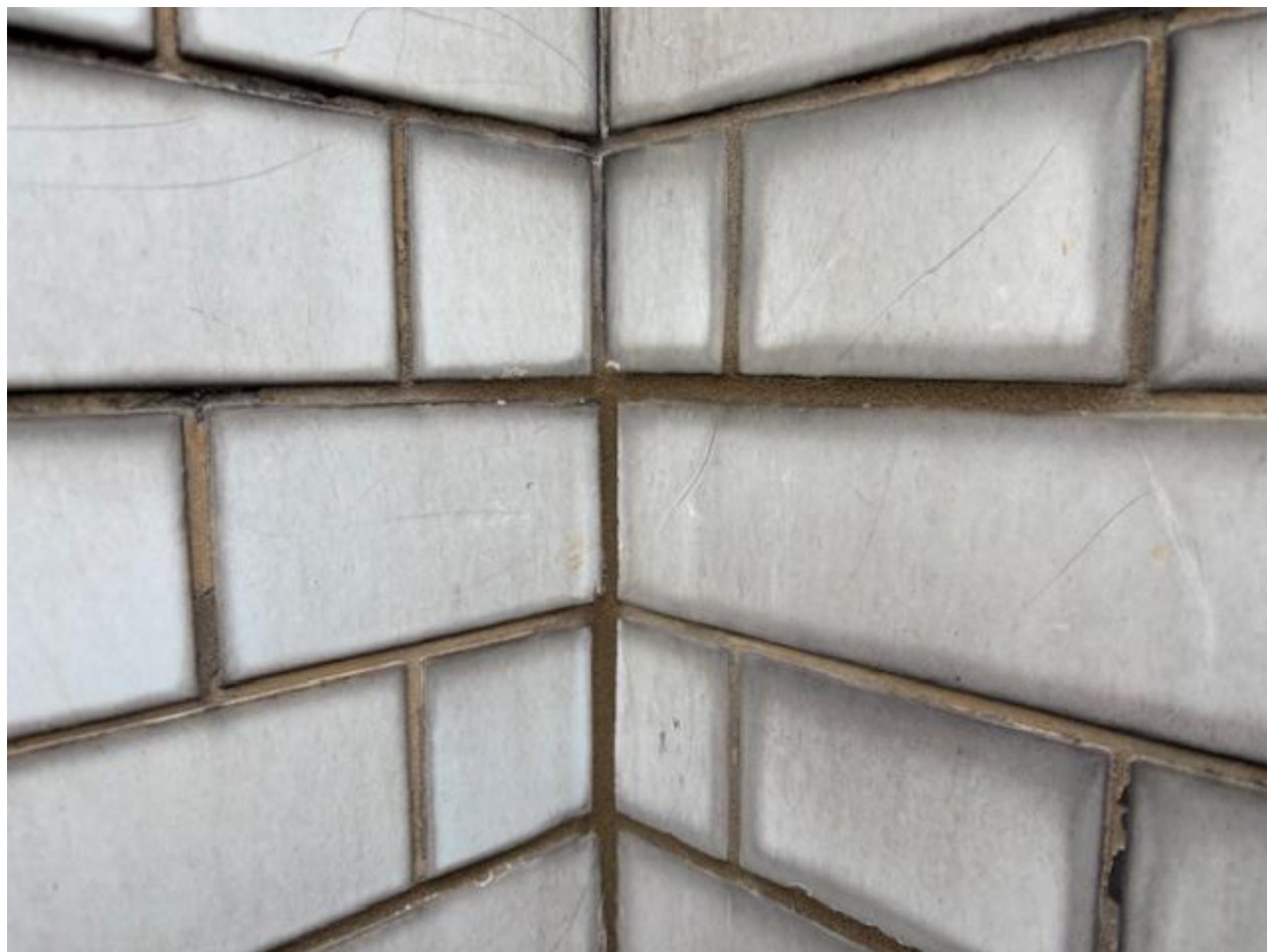
Photo 5. CP ribbon installed and repointed.
