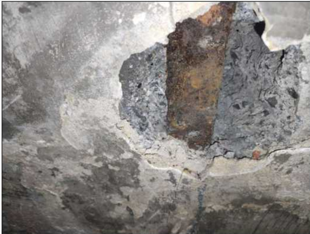
Photo 5: Front flange of joist 3.
