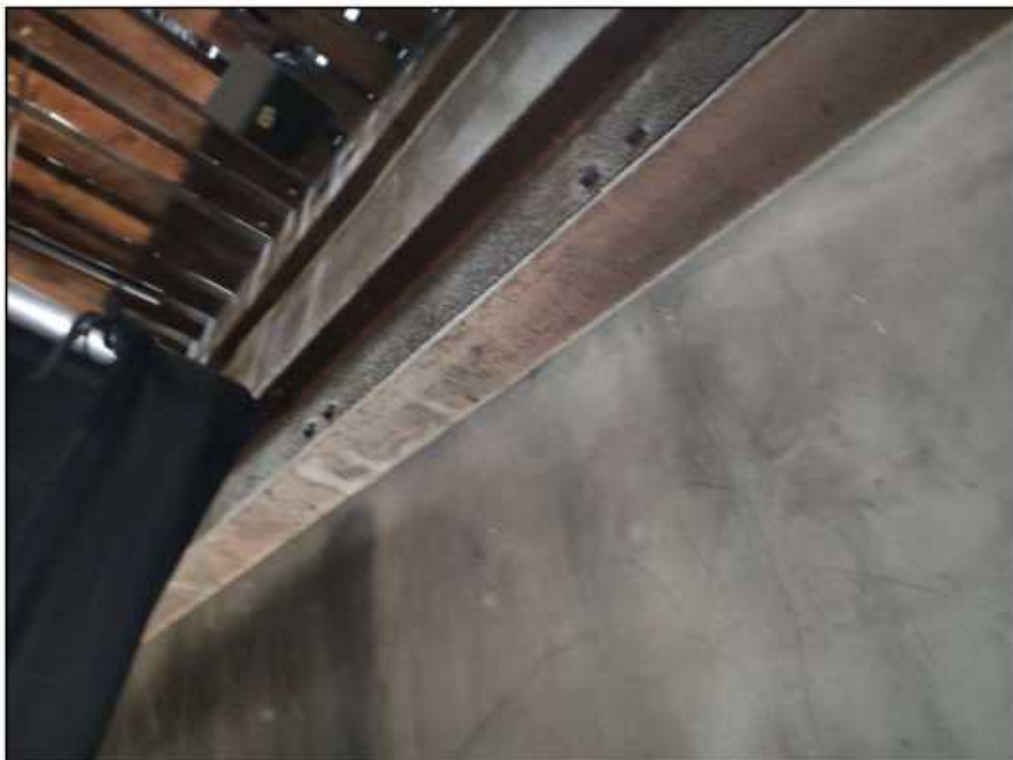
Photo 16: The steel beam towards the top of the sloping section of the wall.
