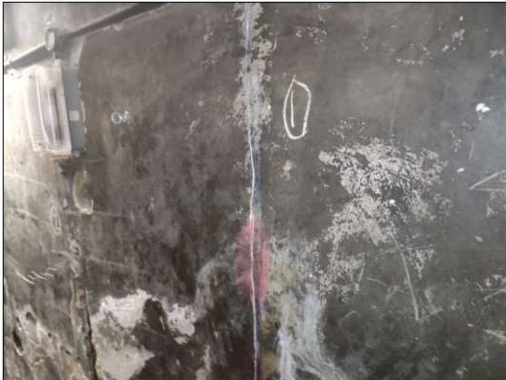
Photo 1: Joist 1, general view before opening-up work. Crayon line indicates position of joist.
