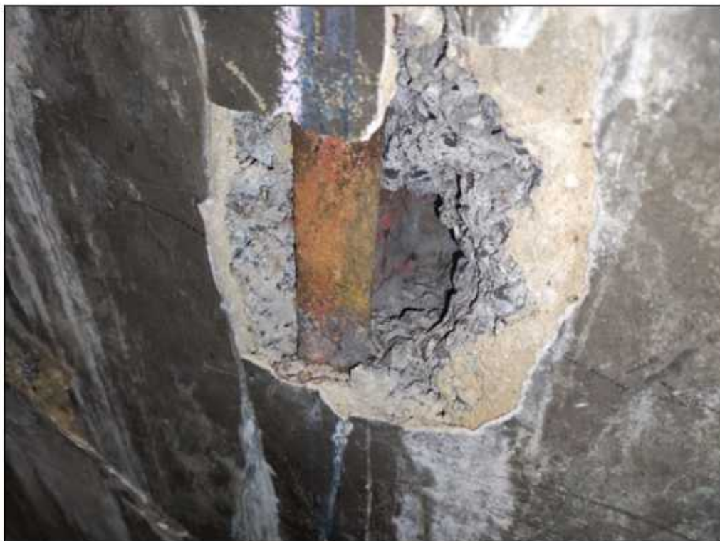
Photo 2: View of the web and front flange of joist 1.
