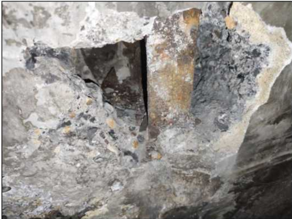
Photo 11: The rear flange at joist 6 exhibits severe corrosion with much of it missing.
