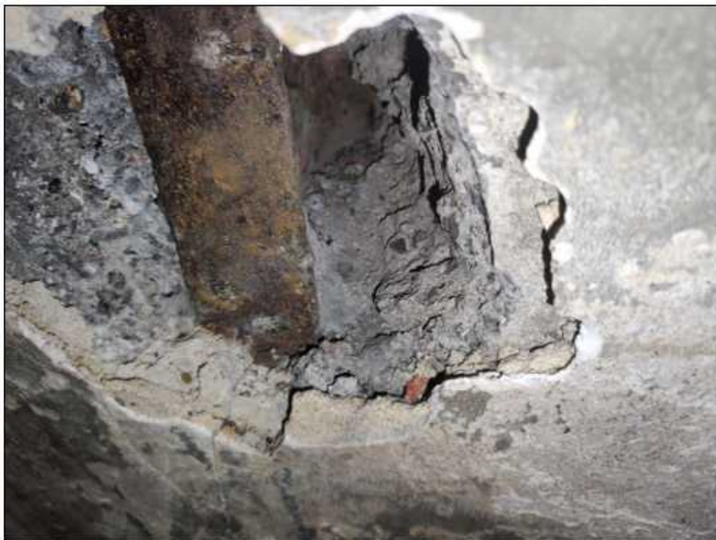
Photo 6: View of the rear flange, web and front flange of joist 3.
