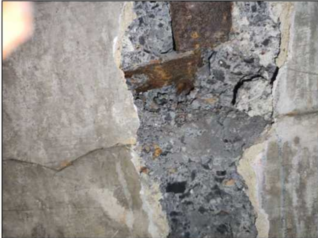
Photo 17: The horizontal steel section attached to joist 2. No brick wall encountered.
