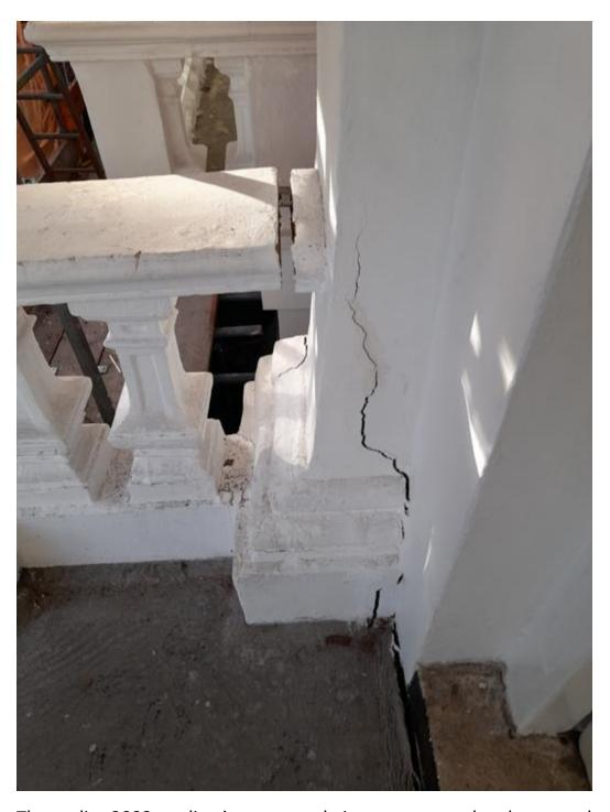
The earlier 2023 application was made in response to the above cracks in the entrance porch to 104 Haverstock Hill which appeared due to the severe summer drought of 2022.
