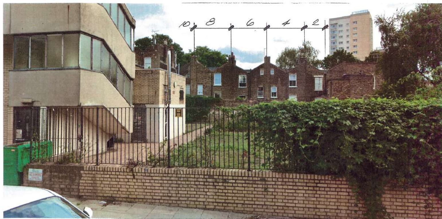
STREET 'REAR VIEW' OFF ALLCROFT ROAD - FROM BASSETT STREET.
