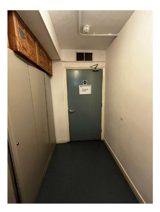
Remove and dispose old door and frame, Fit a new fire doorset with new hardware and archiraves, All factory paint finished
