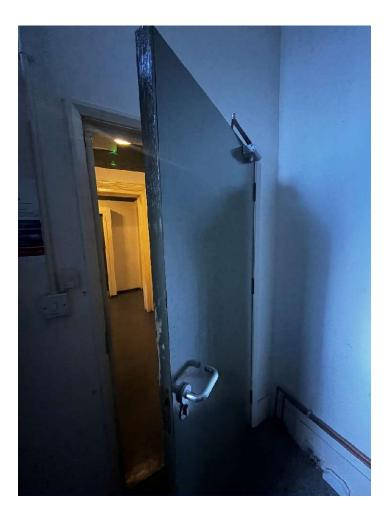
Carry out intumescent paint/paper upgrade works to door in accordance with English Heritage Guidance, allow for rubbing back paint finish applying hardwood fillet to sides of door to square up and fit frame correctly. All works to satisfy the fire engineer to be consultant on the works, repair and make good frame.
