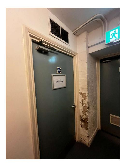
Remove and dispose old door and frame, Fit a new fire doorset with new hardware and architraves, All factory paint finished
