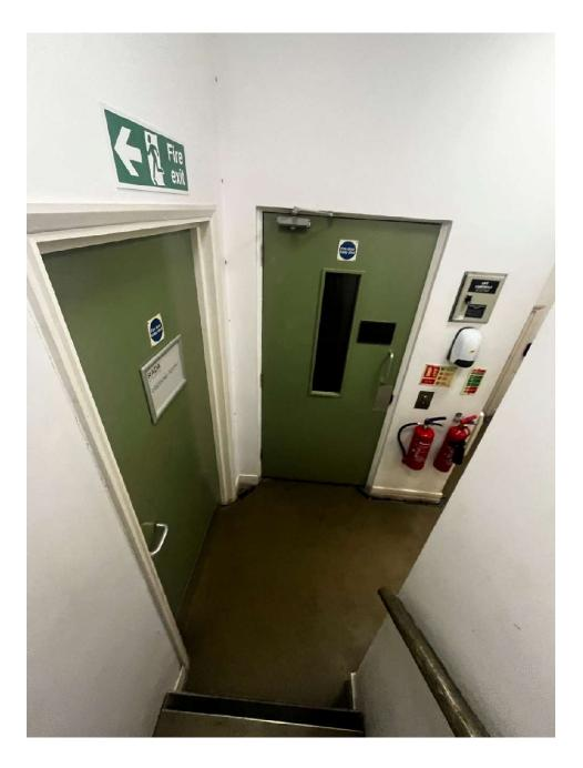
Remove and dispose old door and frame, Fit a new fire doorset with new hardware and archiraves, All factory paint finished
