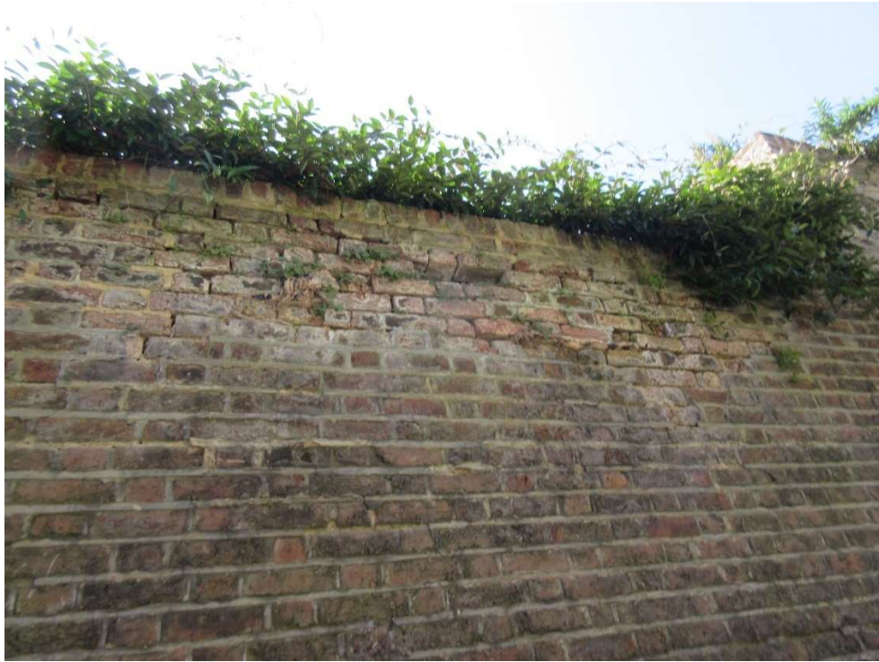
3) Area of brickwork in need of repair and repointing.
