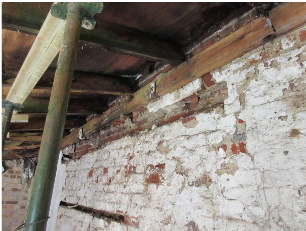
4) On the garden side of the wall, at first floor level (above the gaol), stands a lean-to outbuilding. Water has entered the wallhead and caused its decay. The rotting modern structure is to be rebuilt, like-for-like. Lead capping will be added to the top of the wall to protect the wall from saturation and prevent a recurrence.
