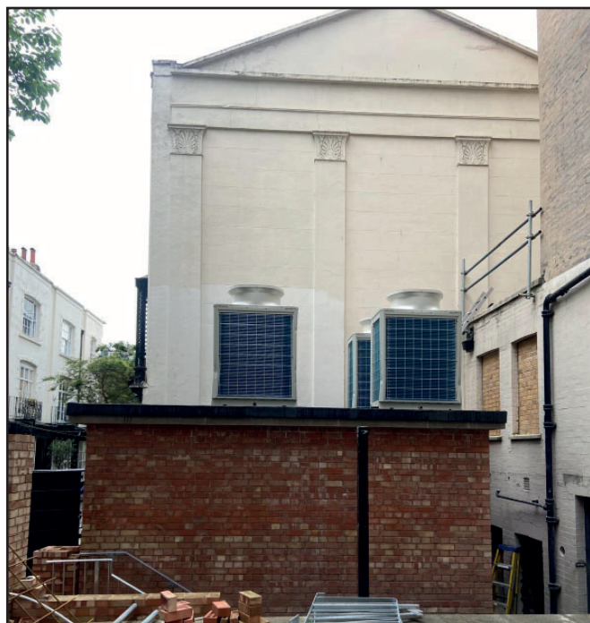
Figs. 11.and 12. As installed ASHPs arrangement (June 2024)
