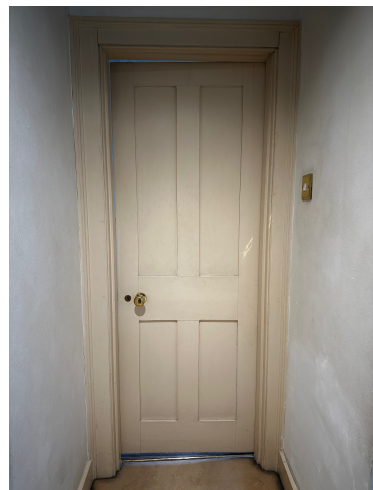
D 1.01 Existing door to bathroom
