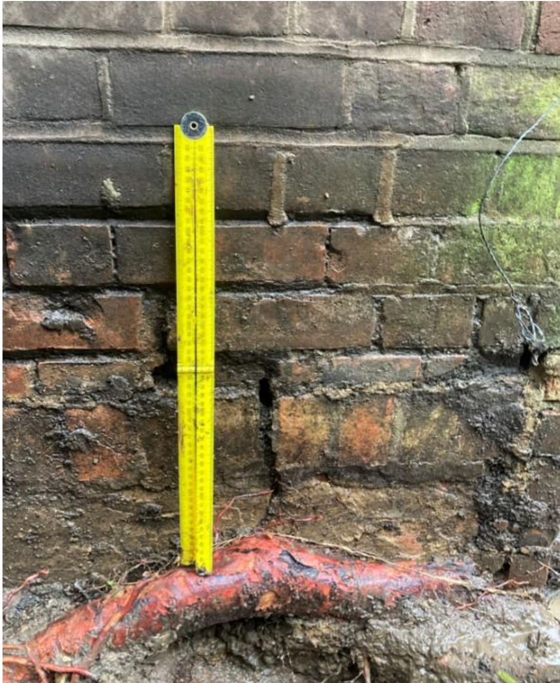
Fig 18: With the tree roots exposed, there is evidence that they are going under the foundations of the listed building.
