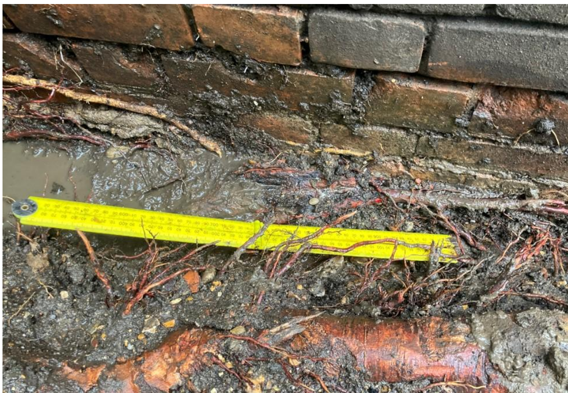
Fig 17: The size of the tree roots relative to the brickwork of the rear wall of the listed building. © SJA Trees 2024
