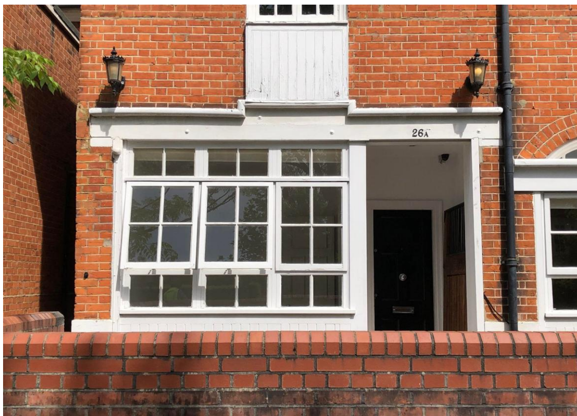
Fig 5: The former vehicle entrance originally had a pair of timber barn style doors, with the lintel being original. The existing door and windows are from the late 20 th Century and of no historic fabric value.
