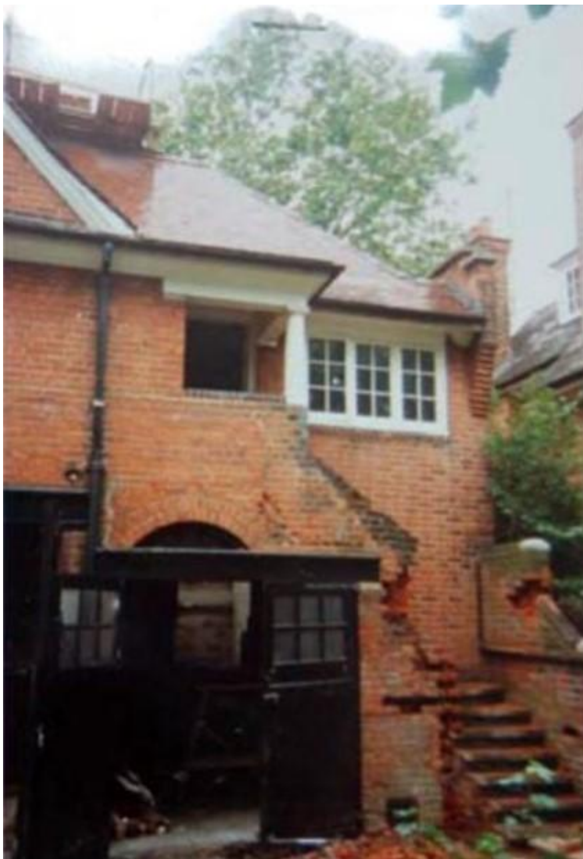
Fig 14: The photo shows the building under conversion in the 1980's with a pair of smaller garage doors in the side opening and the brickwork to the first floor staircase badly damaged and now subsequently rebuilt. © London Borough of Camden 2023
