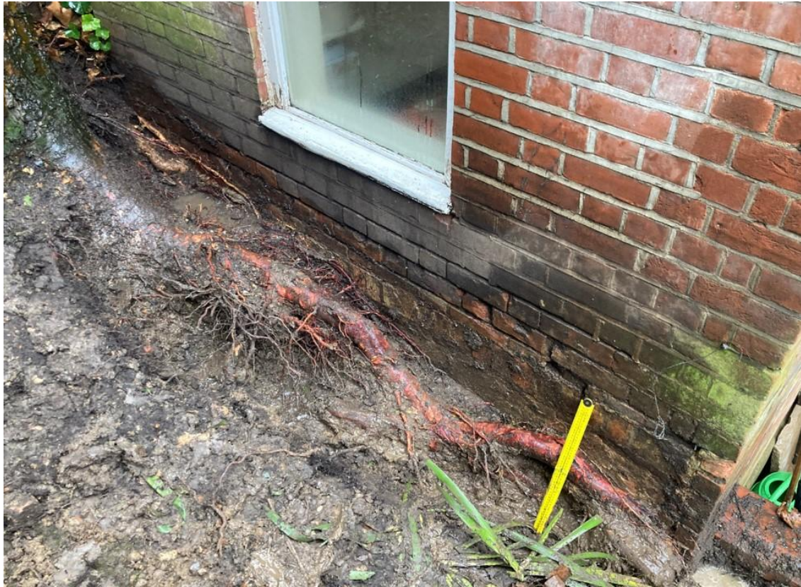
Fig 16: The tree roots are extensive and well established, directly abutting the listed building. © SJA Trees 2024
