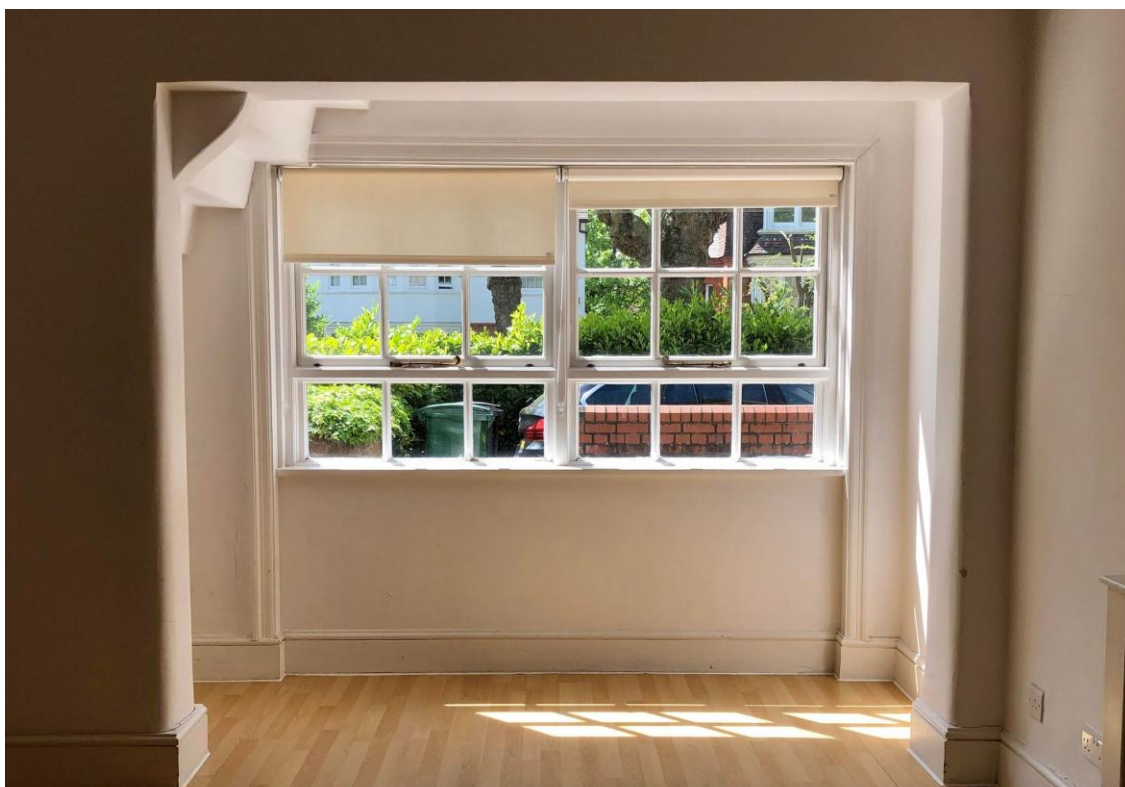
Fig 12: The existing front window does not contain any historic fabric and dates from the late 20 th Century, when the building was converted to a dwelling. Many of the internal features date from this conversion.
