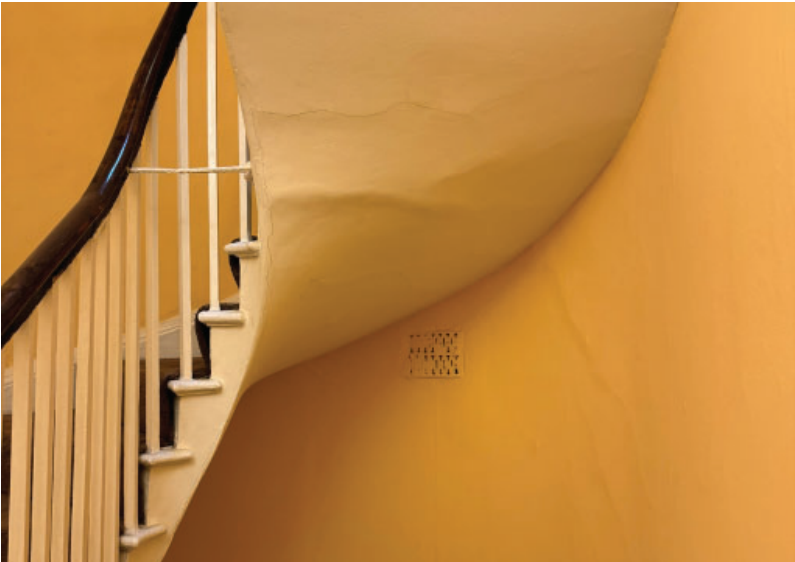
Photo 02 (Above) No.70. Cracking to ceiling and wall below stair.
