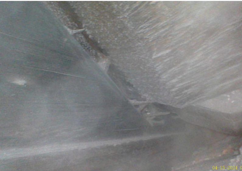
Photo 05 (Above) No.70. Opening of Connection between Outer String and Tread/Riser
