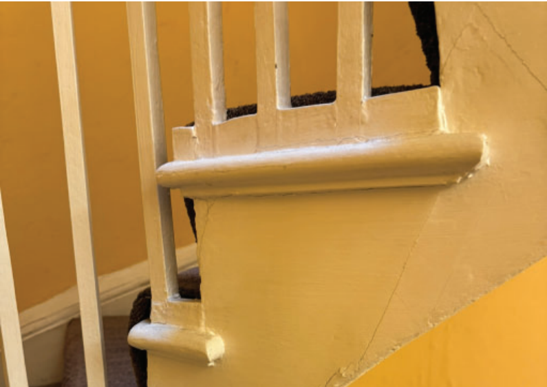
Photo 01 (Above) No.70. Non-original furring piece over the existing tread.
