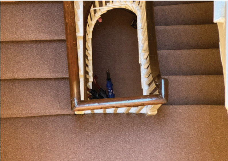
Photo 04 (Above) No.67. Distortion of Balustrade
