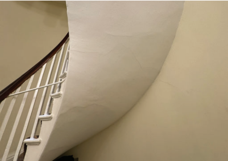
Photo 03 (Above) No.68 Cracking to ceiling and wall below stair.
