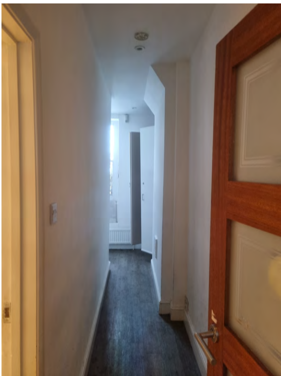
17b Ground floor level corridor looking towards the rear. The corridor is too narrow to form part of a fire escape route.
