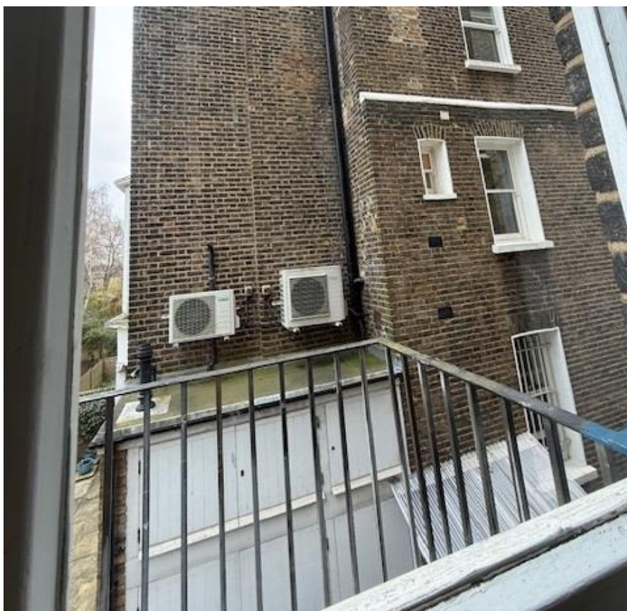
Neighbours wall mounted condensing units (No.38)
