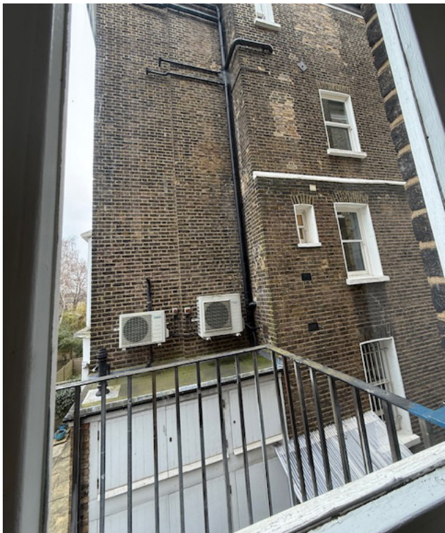
View of No. 38 King Henry's Road Side Elevation Existing External AC Condenser Units (x2)
