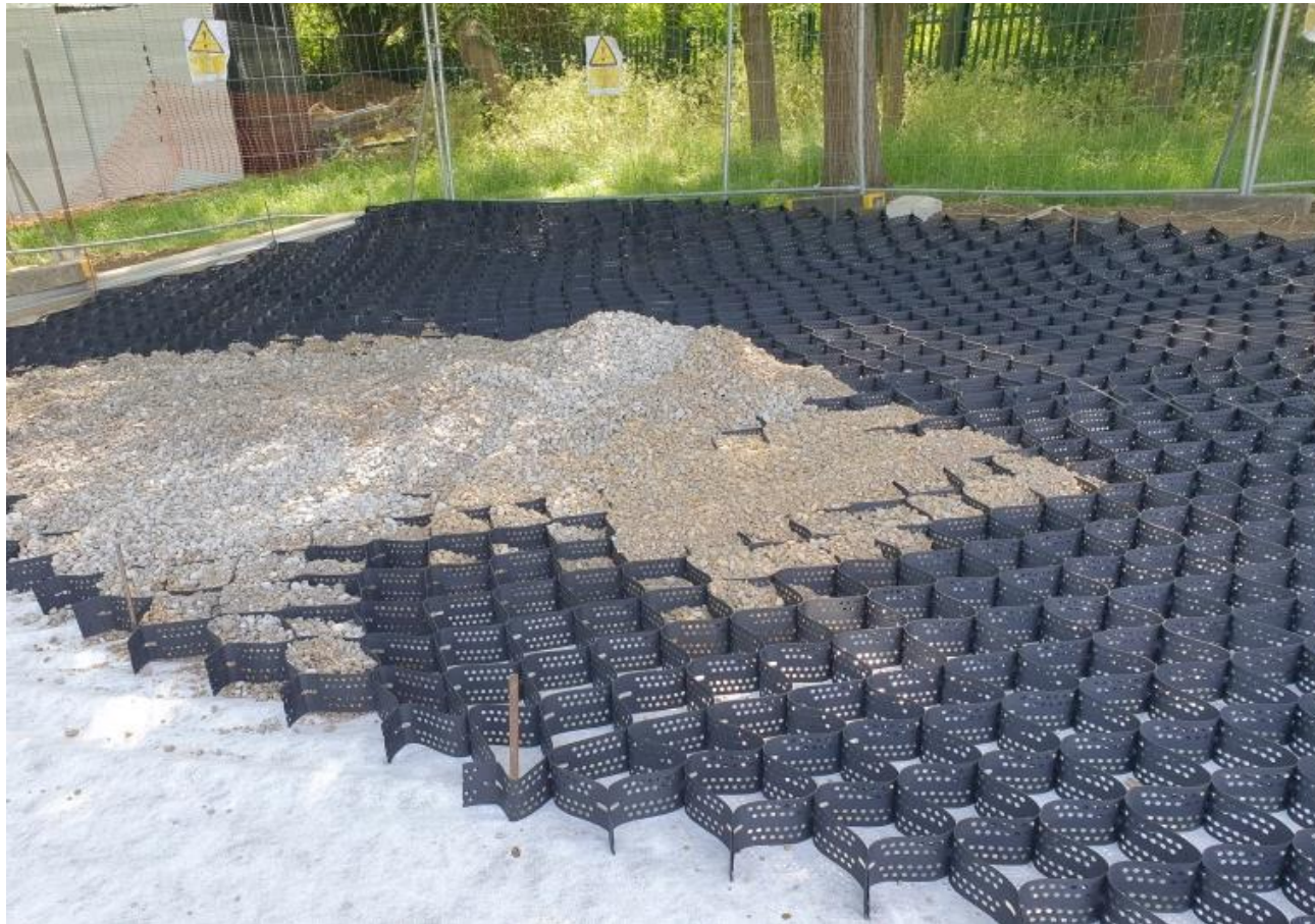
Fig 1: EXAMPLE OF INSTALLATION OF CELLULAR CONFINEMENT SYSTEM
