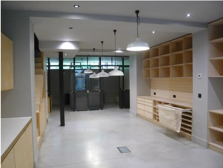
Fig.10 Open-plan layout at lower ground floor – note the nib walls and ceiling beams on former wall lines
