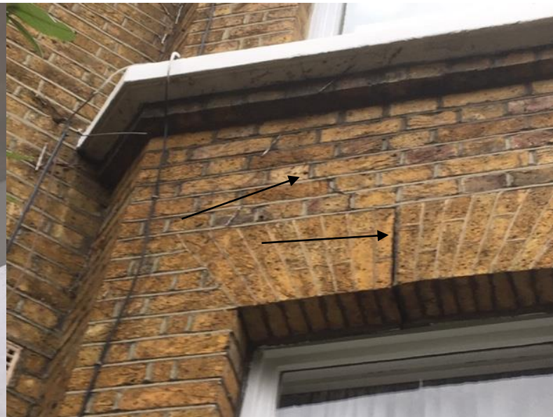
Cracking to bay
