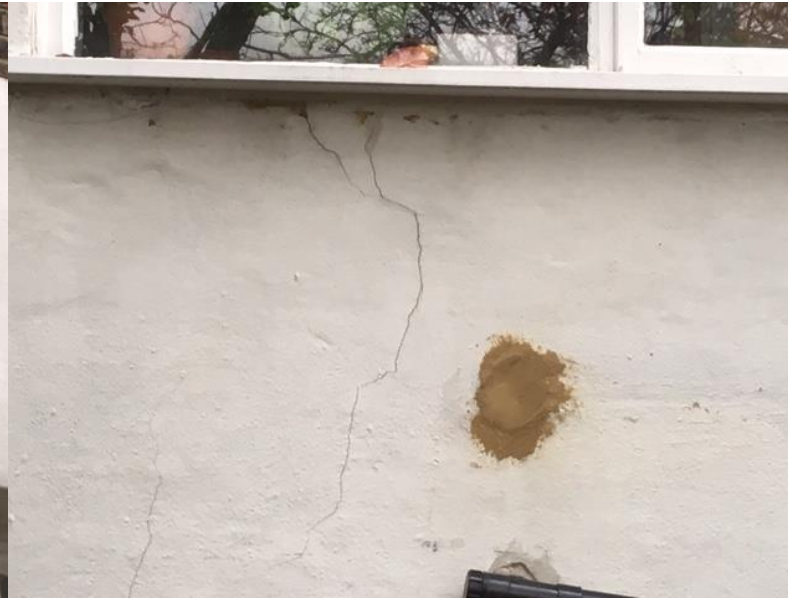
Cracking to rear elevation
