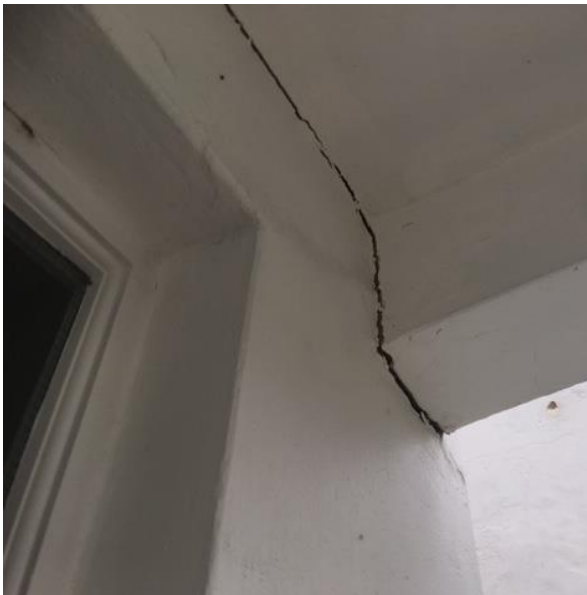
Cracking to porch
