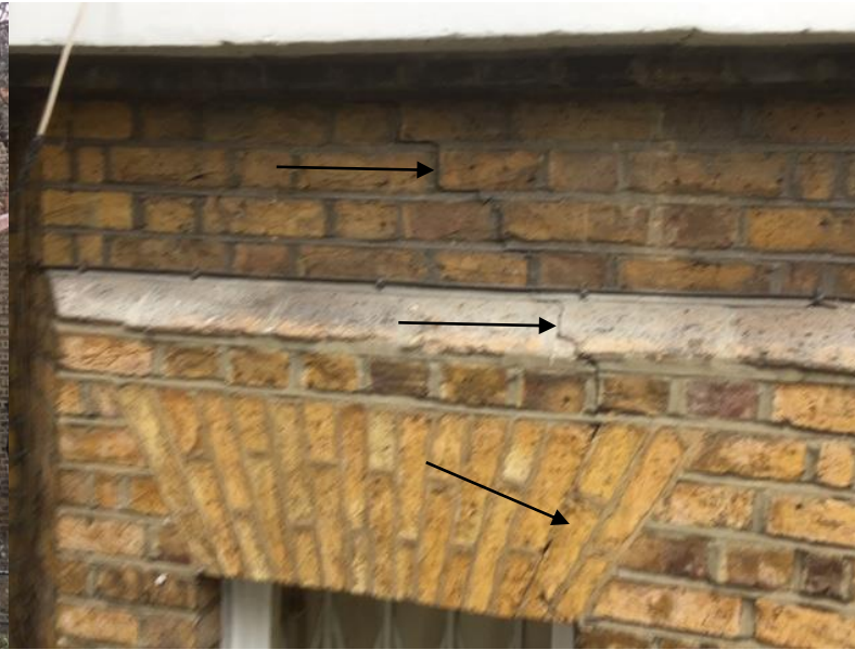
Cracking to bay
