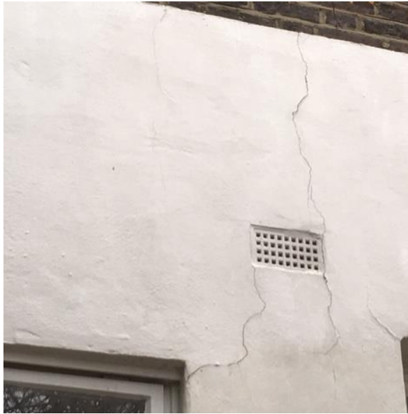
Cracking to rear elevation
