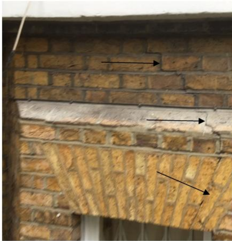
Cracking to bay
