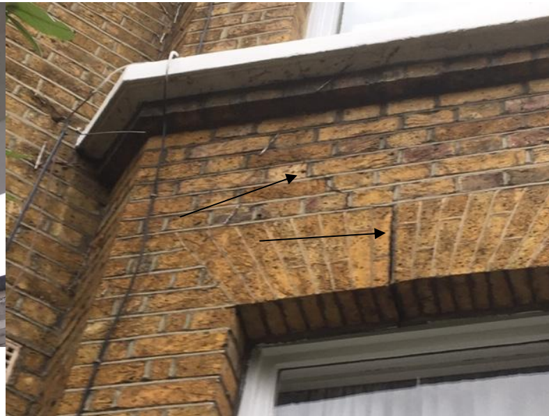
Cracking to bay
