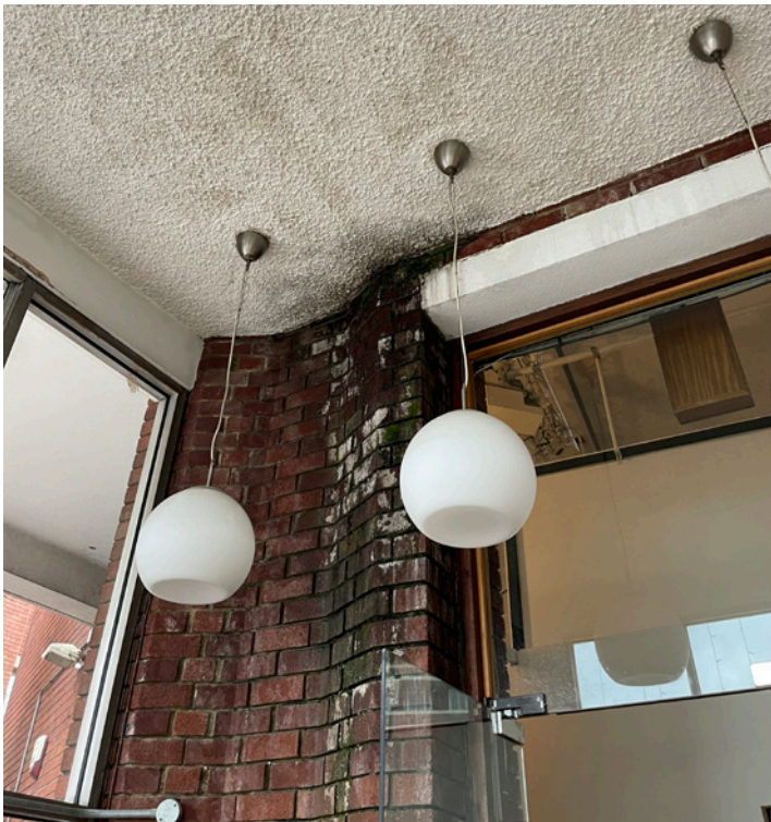
Water ingress from failing roof coverings.
