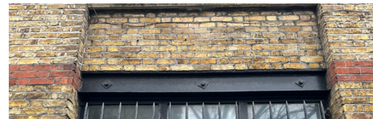
Existing Iron Lintel Retained
