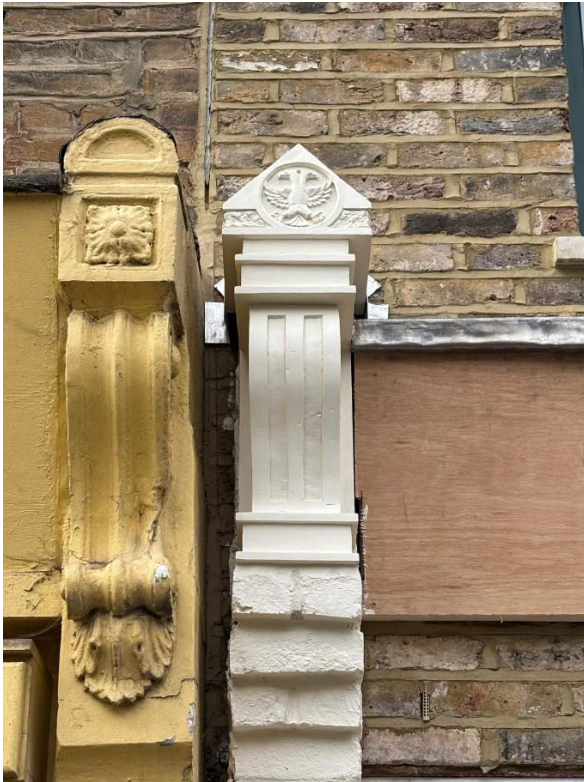
new stone corbel detail to the shop front at no. 147, which is hand carved by a stone masonry craftsman.
