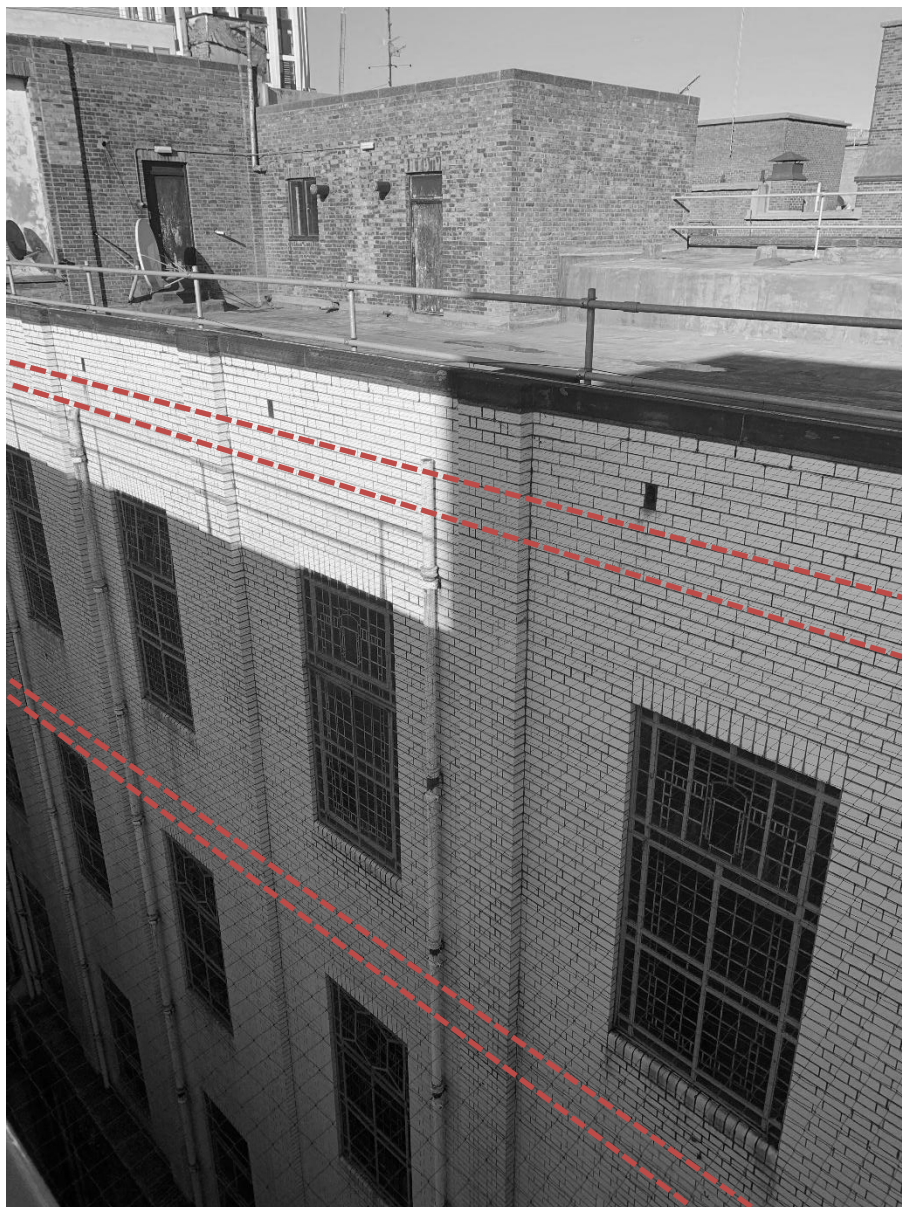
Photograph 3 - Position of anode ribbons for beam protection.
