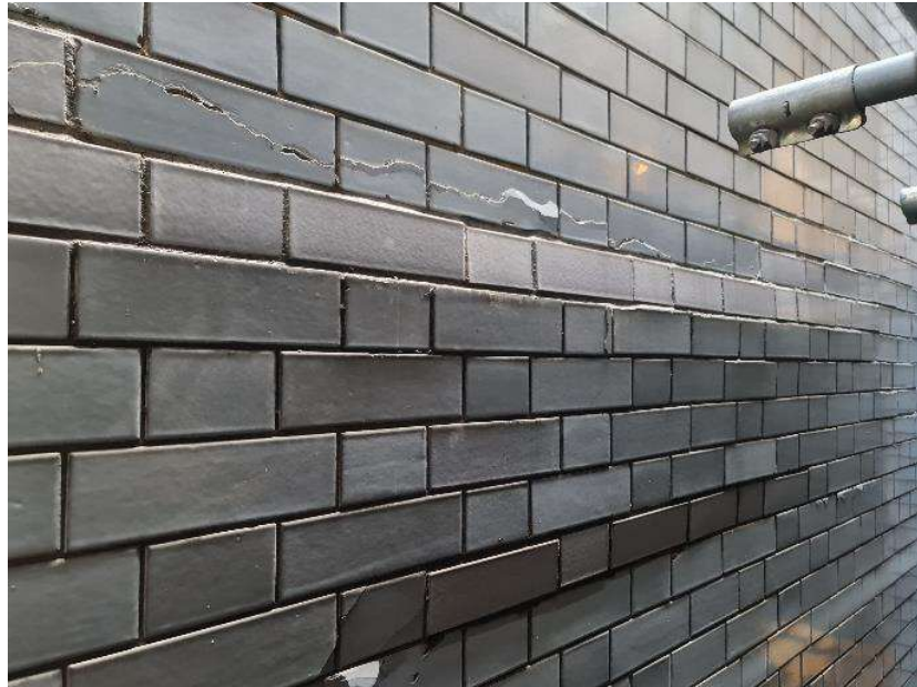
3.0 Example of bulging and cracked brickwork.
