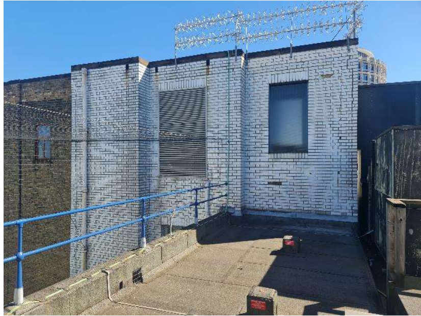
9.0 Brick parapet wall is cracked and leaning inwards.
