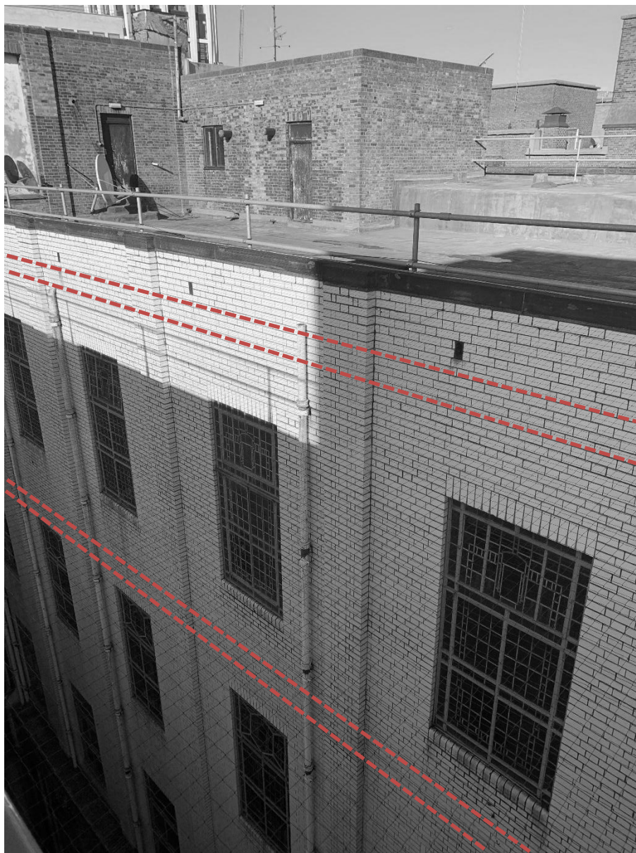
Photograph 3 - Position of anode ribbons for beam protection.
