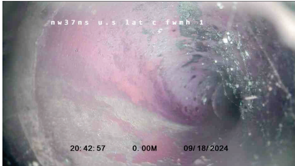
StackY_258e7d10-5cd7-4268-8a6d-db3b72df8407_20240922_124424_257.jpg, 00:00:00, 0.00 m Start node, manhole, reference: FWMH1
