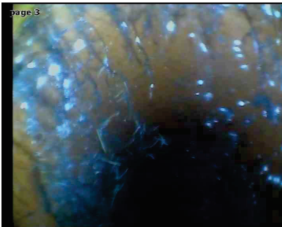
FWMH5X_b43a86fe-5da2-4c1a-85a0-939ac1816a89_20241007_013630_449.jpg, 00:00:14, 0.60 m Roots, fine, start
