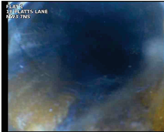
FWMH4X_c8c40d6b-469b-4a22-bcc3-93ee2a049102_20241007_013123_193.jpg, 00:00:00, 0.00 m Start node, manhole, reference: FWMH4
