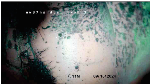
6d2dfc35-97b3-4dc0-83ae-87758a451ba8.png, 00:00:35, 7.11 m Line deviates down
