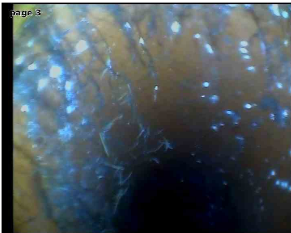
FWMH5X_b43a86fe-5da2-4c1a-85a0-939ac1816a89_20241007_013630_449.jpg, 00:00:14, 0.60 m Roots, fine, start
