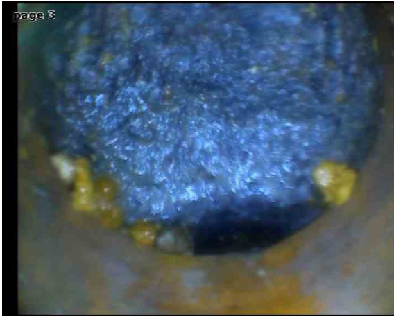
FWMH5X_da81ad58-43de-48ab-ac0c-af8977441448_20241007_013825_178.jpg, 00:00:53, 7.90 m Roots, mass, 90% cross-sectional area loss
