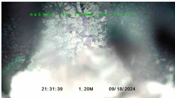
87a894b7-0156-42bd-9139-5314e2be234a.png, 00:00:09, 1.20 m Settled deposits, fine, 15% cross-sectional area loss
