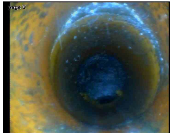
FWMH5X_8aaea2d5-d64c-4bc7-8aee-dac7876d4129_20241007_013734_189.jpg, 00:00:36, 6.00 m Roots, fine at joint
