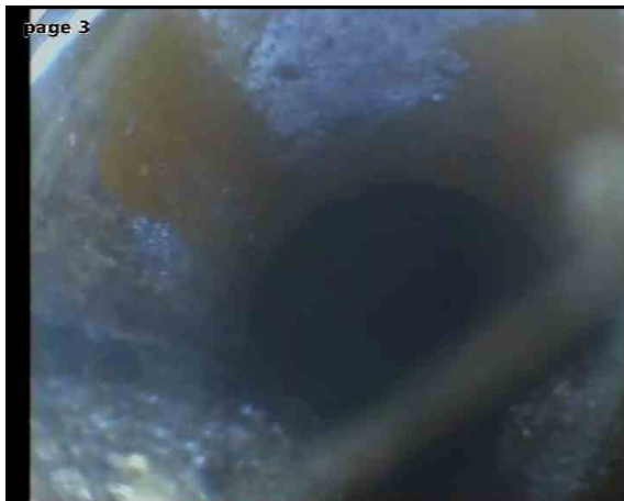
FWMH4X_94a2c97c-eaee-4857-9370-c830deef467_20241007_013211_693.jpg, 00:00:17, 0.00 m Attached deposits, grease from 12 o'clock to 12 o'clock, 15% cross-sectional area loss, start
