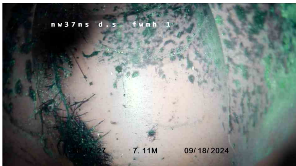
6d2dfc35-97b3-4dc0-83ae-87758a451ba8.png, 00:00:35, 7.11 m Line deviates down
