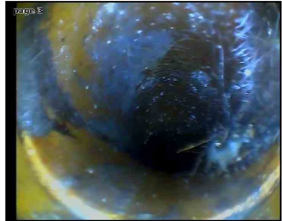
FWMH5X_4012fe3c-2693-4359-b224-8d47829c168f_20241007_013558_121.jpg, 00:00:11, 0.50 m Roots, mass at joint, 20% cross-sectional area loss
