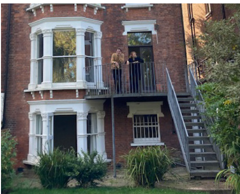
Existing metal stair and terrace accessed from the first floor rear
