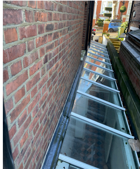
Existing PVC fixed roof light, issues with leaking and unsatisfactory detailing around downpipes.
