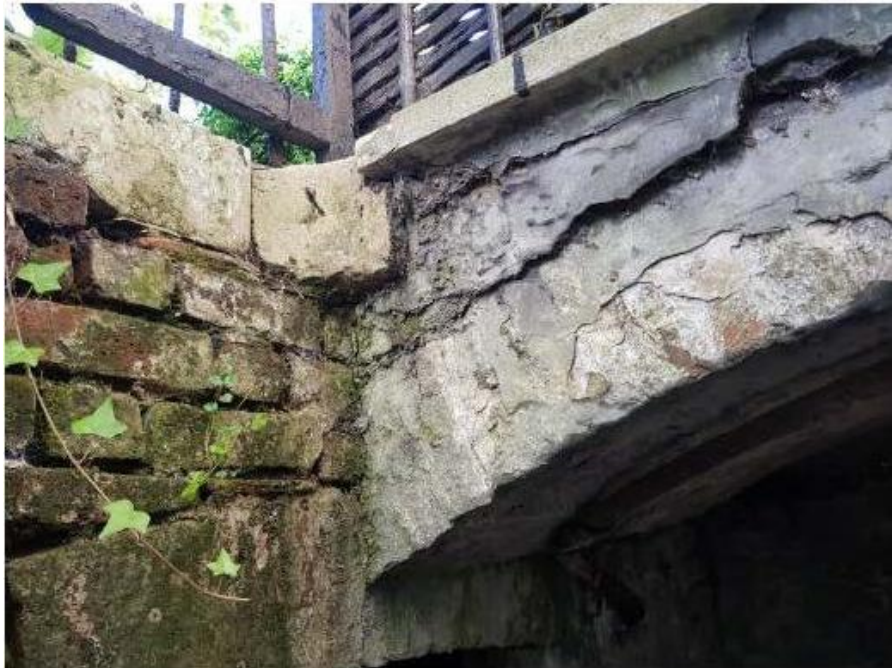
View C- cracked brickwork below balustrade and above arch
