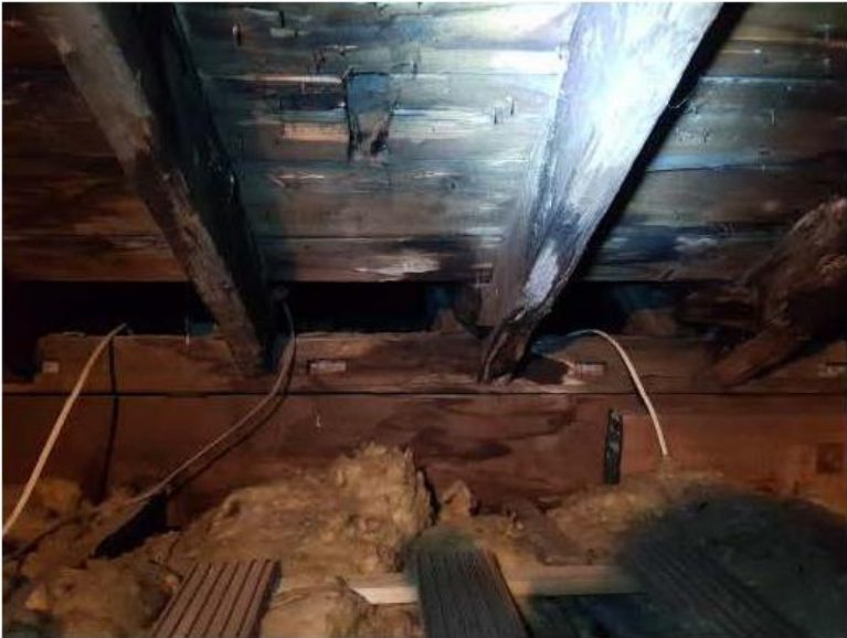
Wet rot to ends of rafters and wall plate to be cut out, and new timber of same section spliced in
