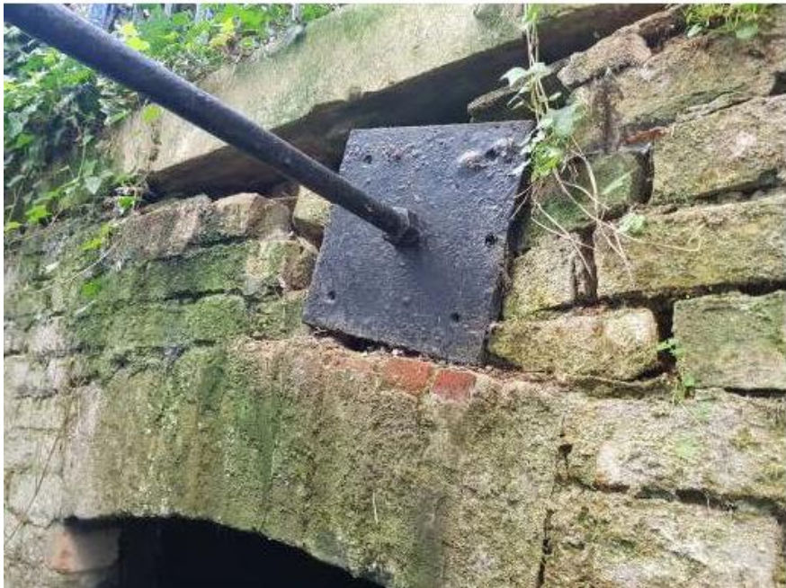
View B- brick arch has failed and joints in brickwork have opened up
