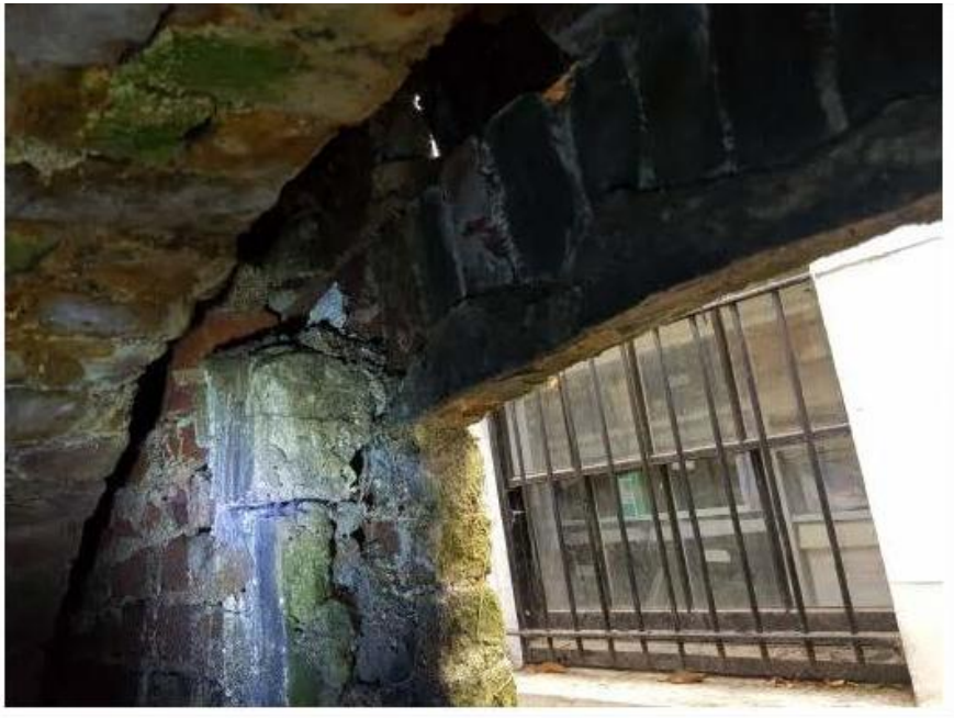
View A-joint between front wall and vault opened up and brick arch failing
