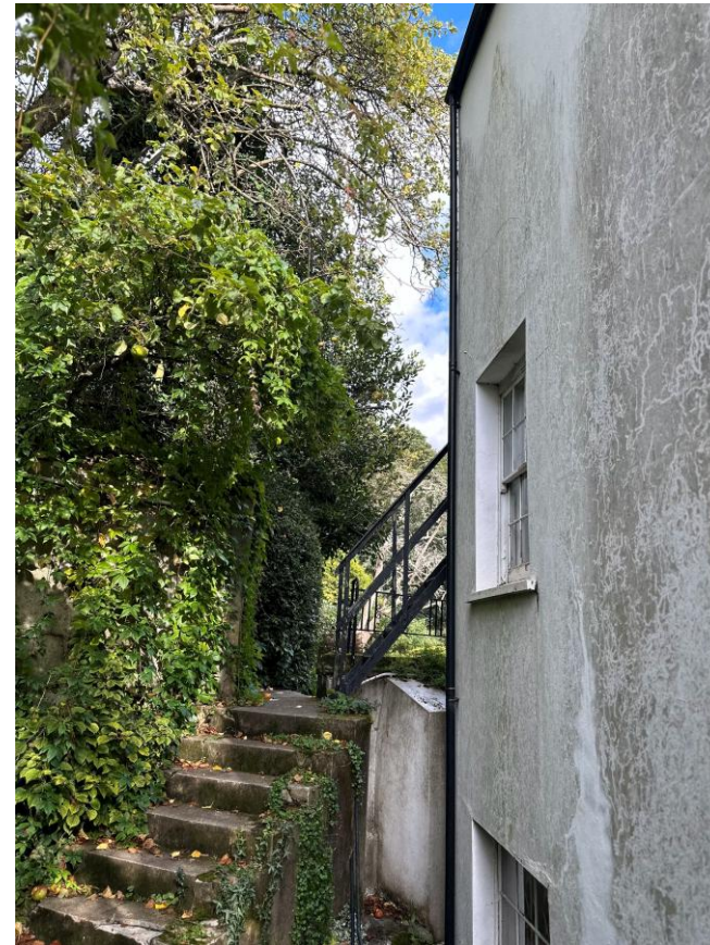
Render cracking and crazing
