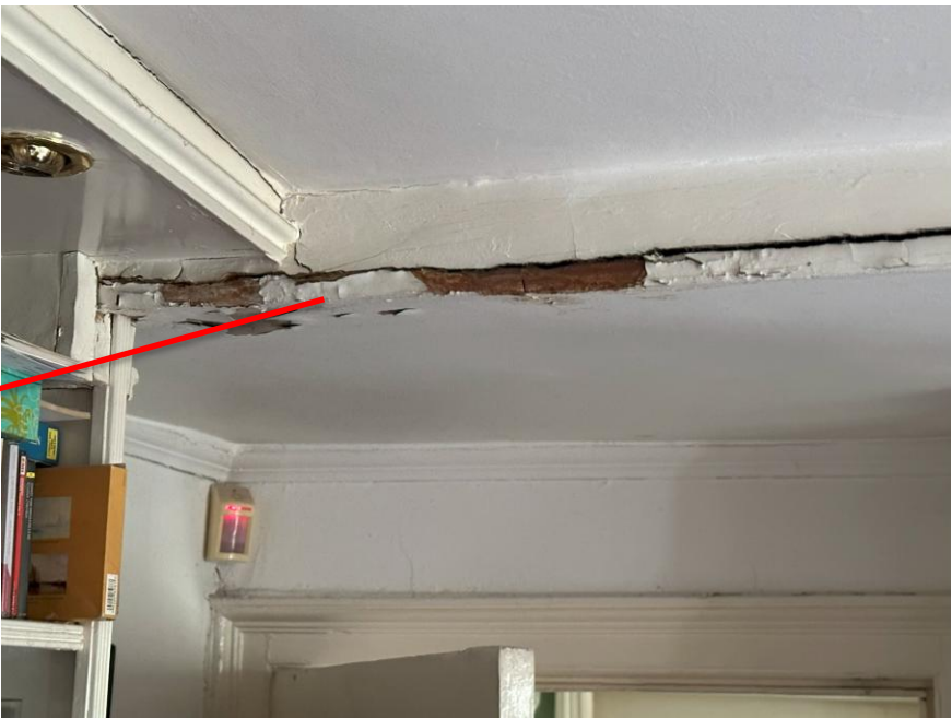
Damp coming through second-floor beam from leaking roof.
