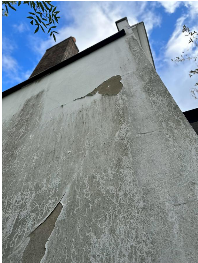
Render cracking and detaching from sub-base
