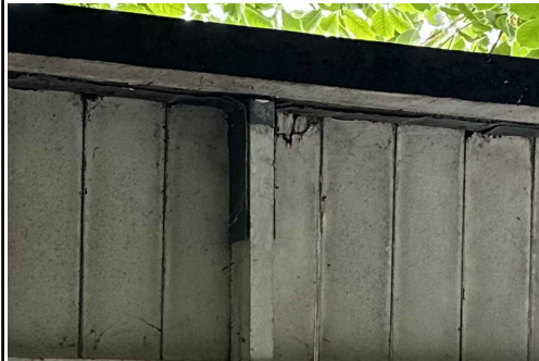
TIMBER JOISTS ROTTED AND SOME BOARDS REQUIRING REPLACEMENT TO BALCONY.
