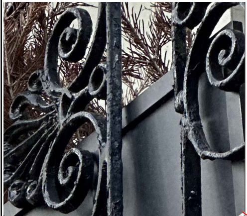
VERTICAL ELEMENTS CORRODED AND JOINTS BROKEN
