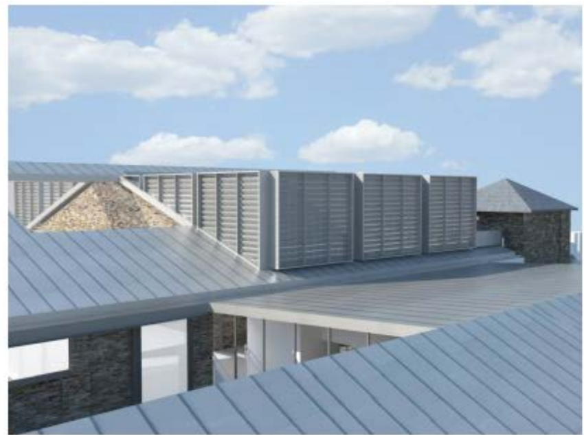
Plant dormer to MGS roof, off set from eaves and below roof ridge
