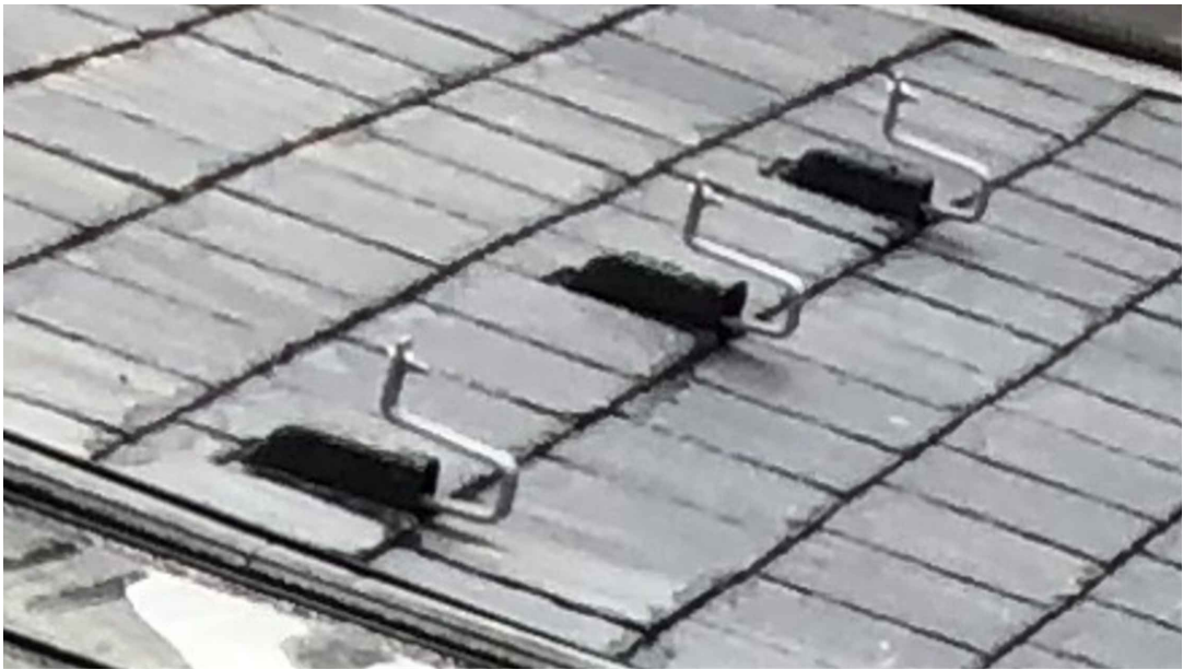
Typical Roof Hook
