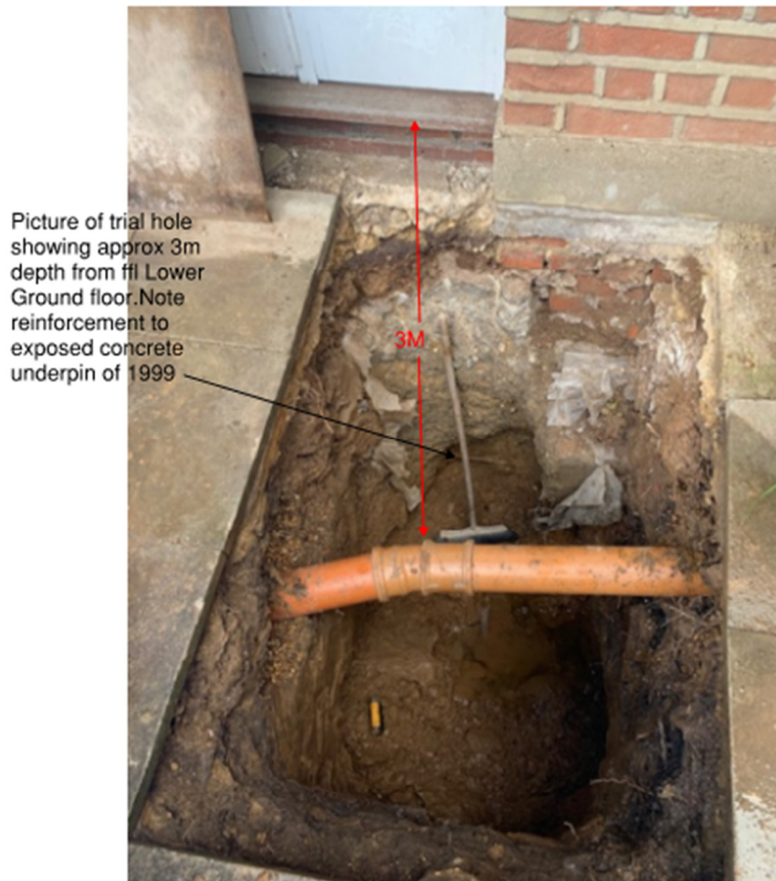
Recent trial pit Underpin exposure of 1999 whole building underpin 9 th Nov 2023.
