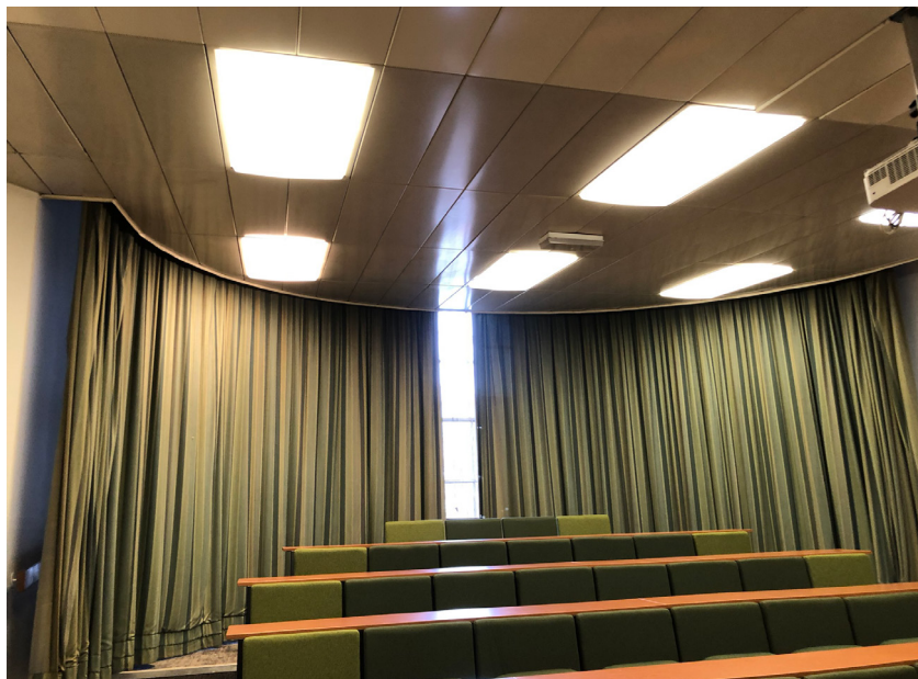
Fig. 13: The curtains covering the windows – difficult to move and usually kept closed. Poor ceiling condition above
