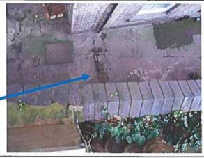
In addition to this the neighbouring footpath has suffered direct damage from tree roots as shown in the photograph opposite which could form a trip hazard.
