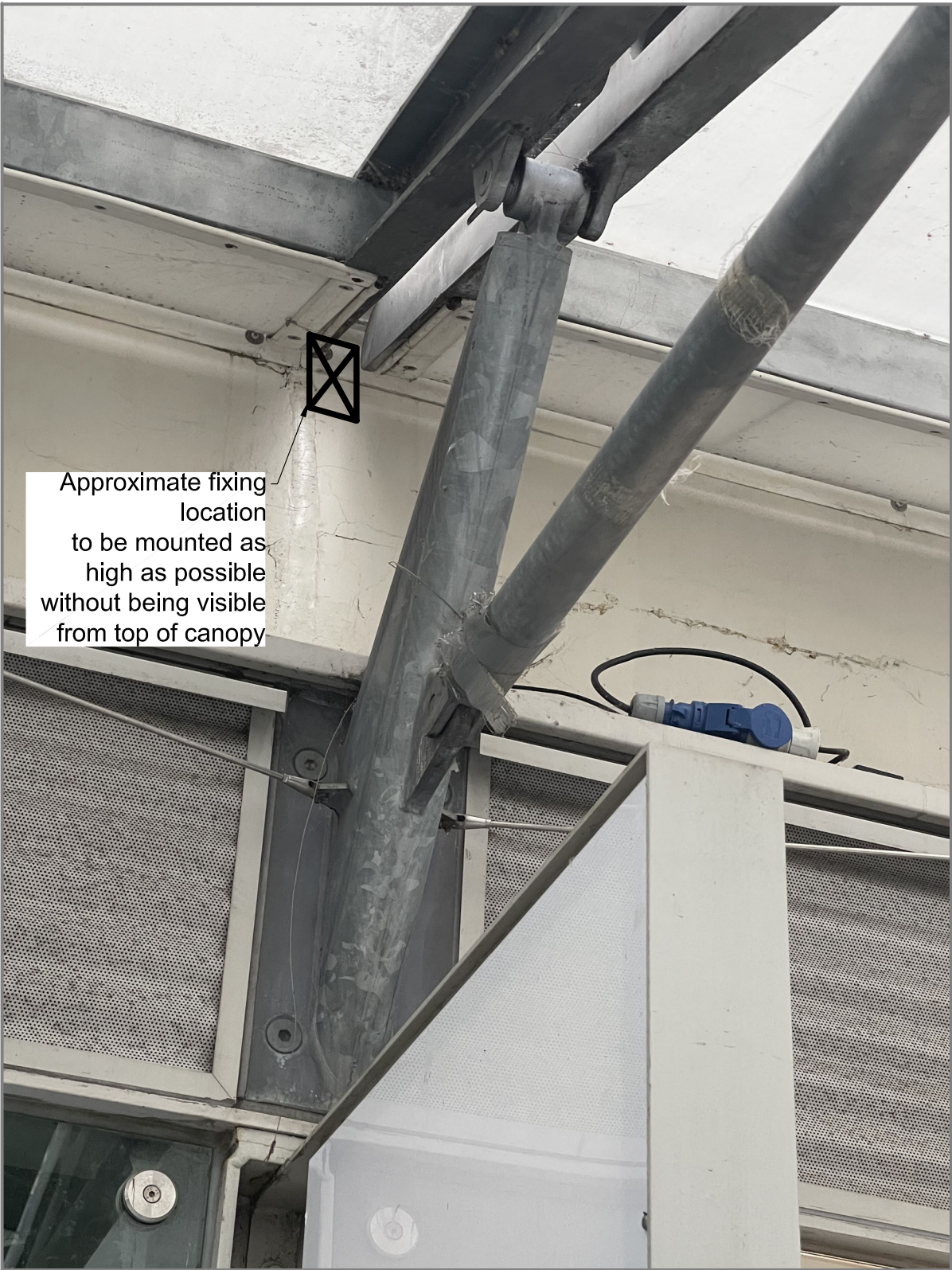
Festoon lighting fixing
