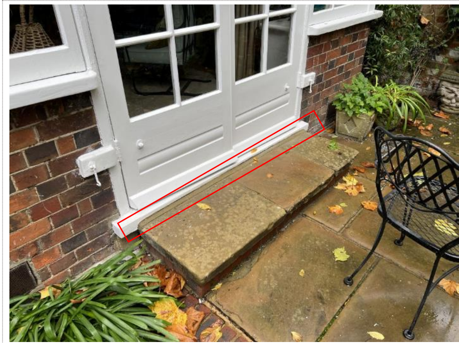
Plate 3. Displaced step now filled with grout.
