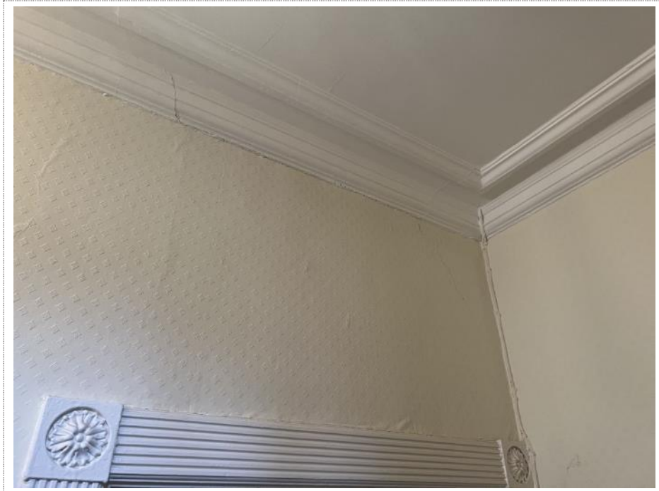
Plate 7. Cracking to wall in hallway.
