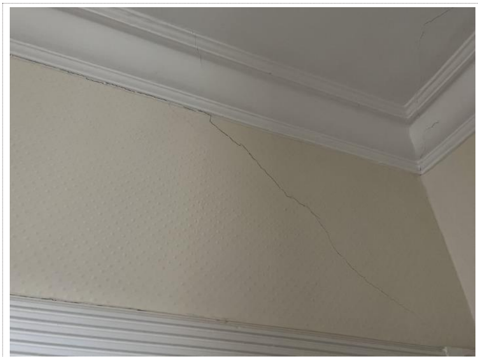
Plate 12. Further view of cracking.
