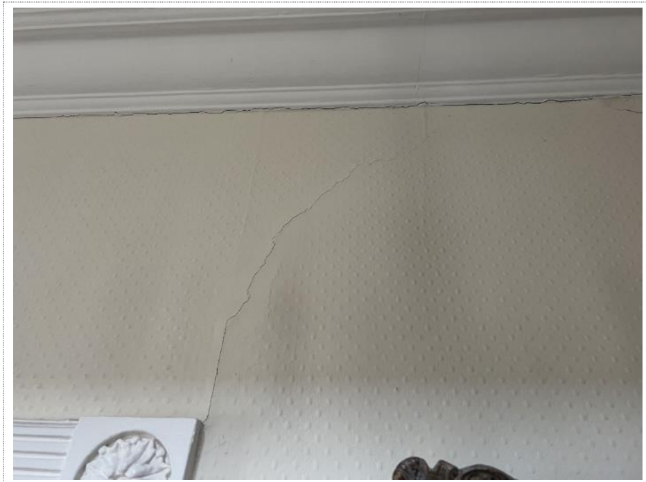
Plate 13. Cracking in hall above door to front bedroom.
