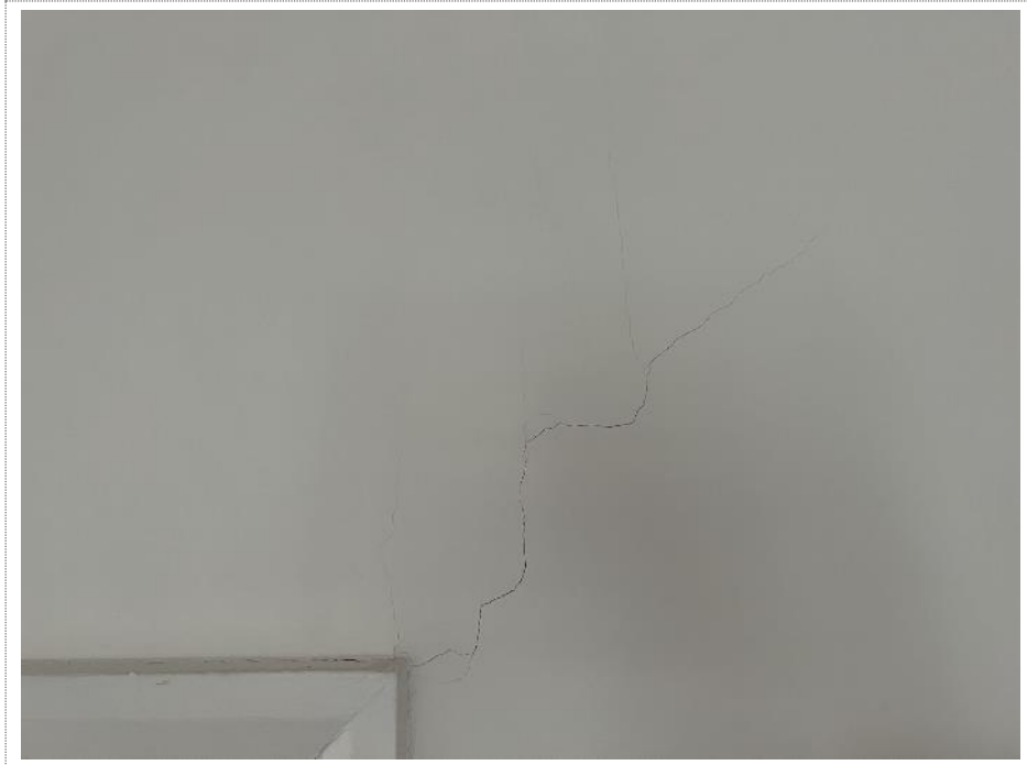
Plate 21. General condition of cracking at second floor level.
