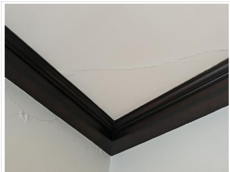
Plate 6. Cracking to ceiling in living room.
