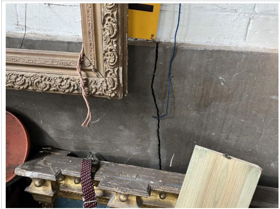
Plate 17. Vertical crack in garage.
