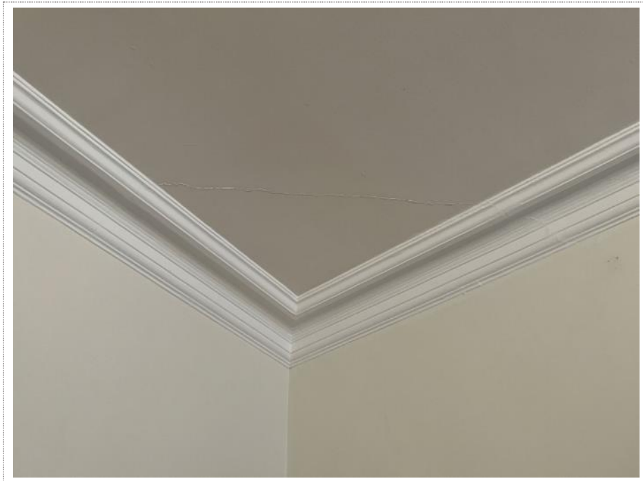
Plate 19. Evidence of existing cracking.
