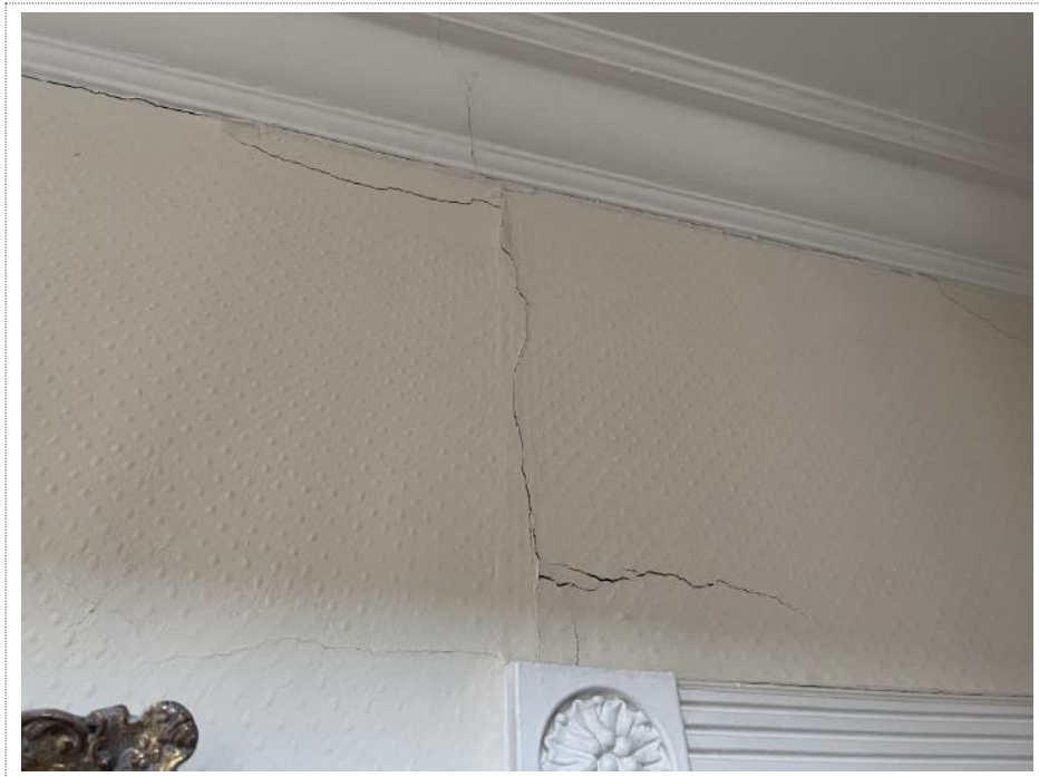
Plate 11. Cracking to landing at FF level.
