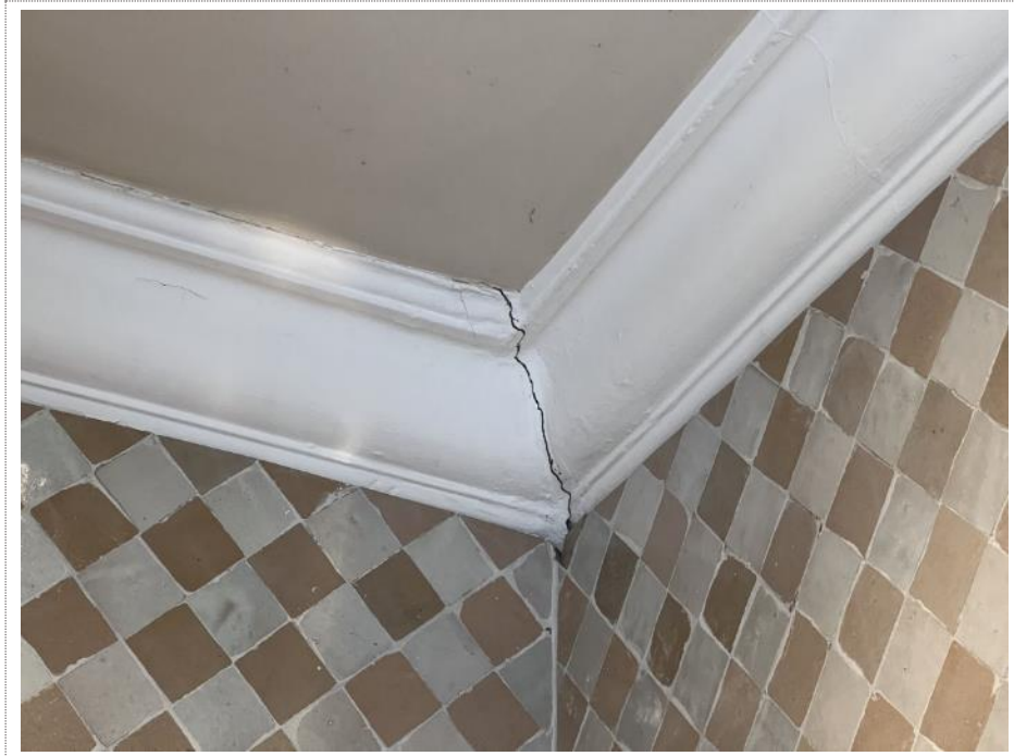
Plate 15. Corner cracking to ensuite.
