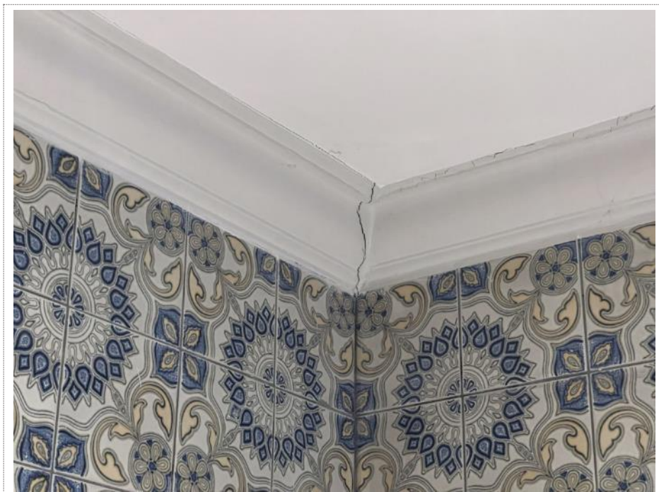
Plate 16. Corner cracking to main bathroom.
