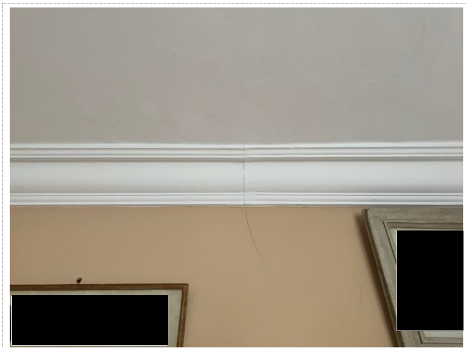
Plate 20. Hairline cracking to coving in office.
