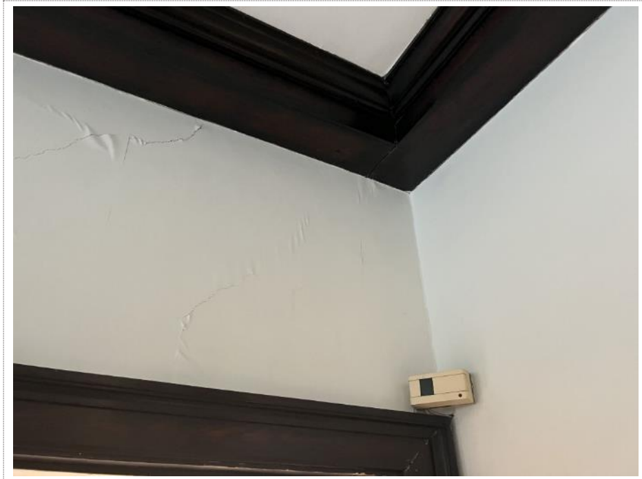
Plate 5. High level cracking to wall in living room.
