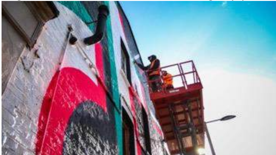
Figure 6 - Use of scissor lift in accordance with highways permit
