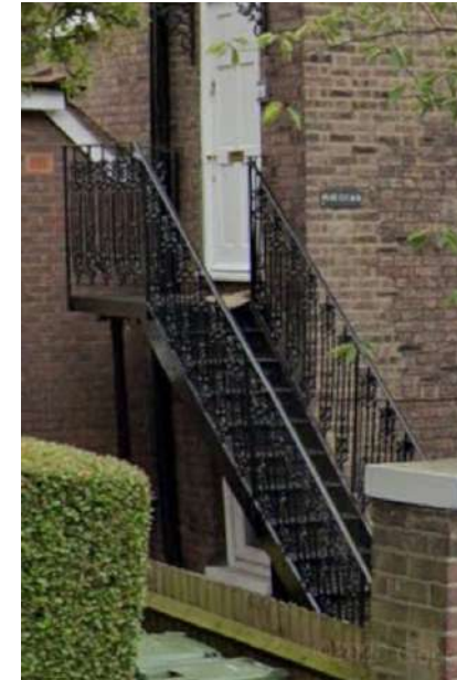
Edwardian railing for cast iron stair leading to no 12b. The railing is painted black.
