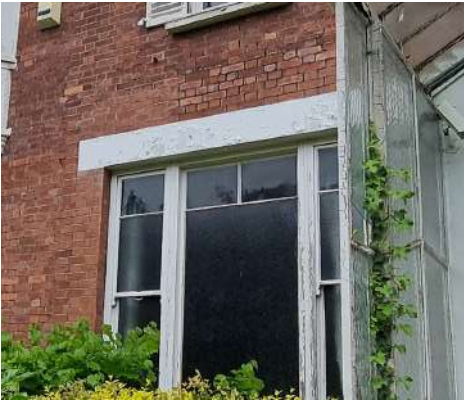
Original brick lintel above window by entrance replaced with modern concrete lintel.
