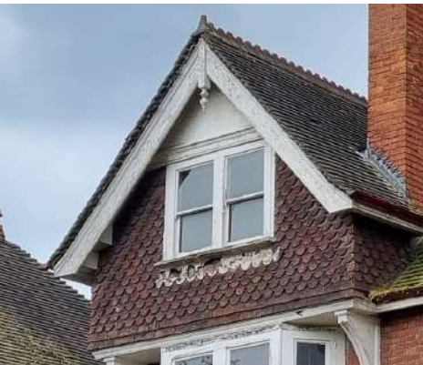
Clay tiles to bay window in need of repair and clean.
