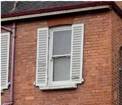
Gauged brick lintels over windows. Timber shutters to sash windows.
