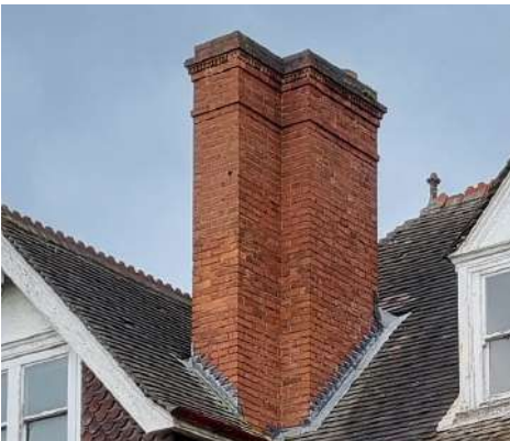
Arts & Crafts chimney flues, in good shape, with flaunching and leadwork needing to be redone.
