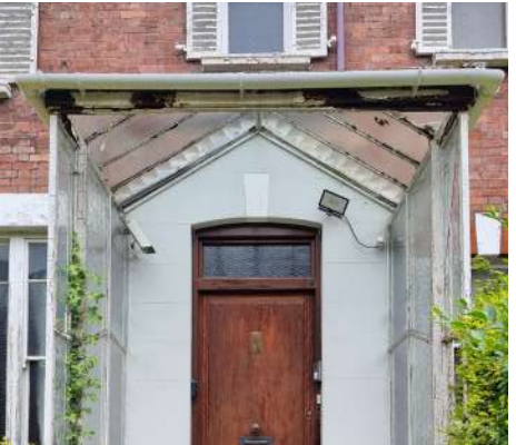
Modern canopy over entrance, to replace feature portico. Brickwalls rendered over, hiding brick lintel.
