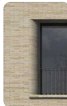
Curved brick reveal in same tonal colours as the rest of the extension.
