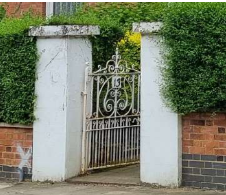
Both pilasters either side of pedestrian entrance have been rendered over with modern material, hiding feature brickwork.
