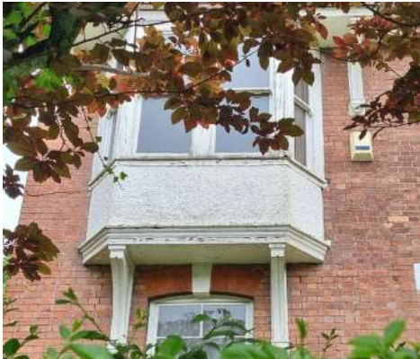
Plaster work to 1F bay window missing, assumed to be covered by modern render.
