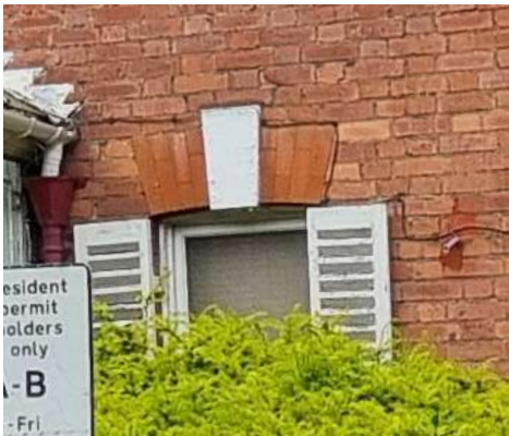
Floral key stone to window lintels missing - assumed either covered in modern render or replaced with modern material.
