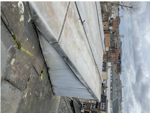
Photograph showing side cheeks to dormer
